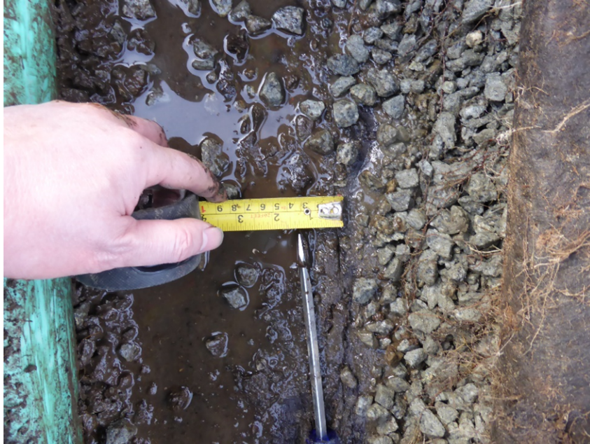
Photo 1: Typical condition at Tests #1 and 2 (except for expansion joint width)
