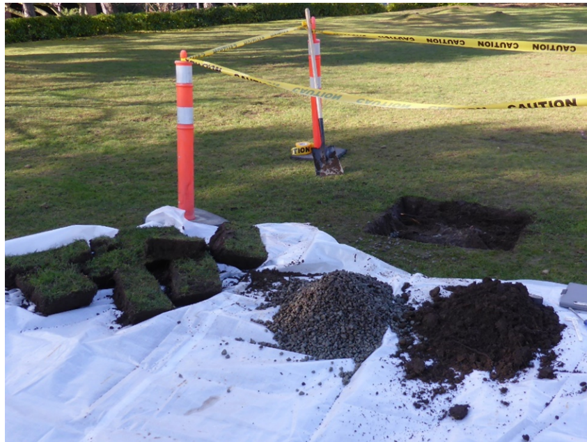
Photo 2: Typical landscaping materials at Tests #1 and #2
