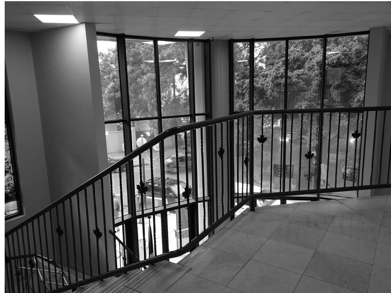
REFERENCE IMAGE FOR DEMOLITION: HANDRAIL TO BE REMOVED / CAP AT TOP OF STAIR
