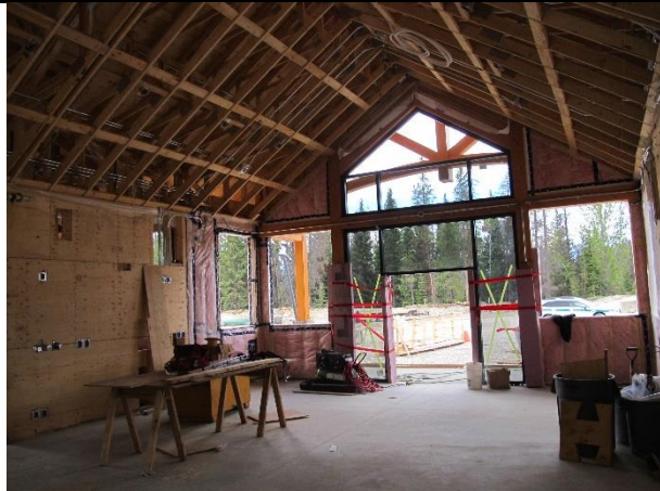
Roof Structure during construction
