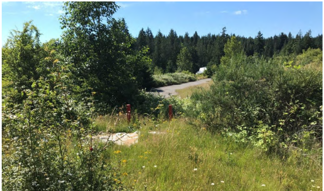
Photograph 8: View of Excavation 2 area, facing southeast.
