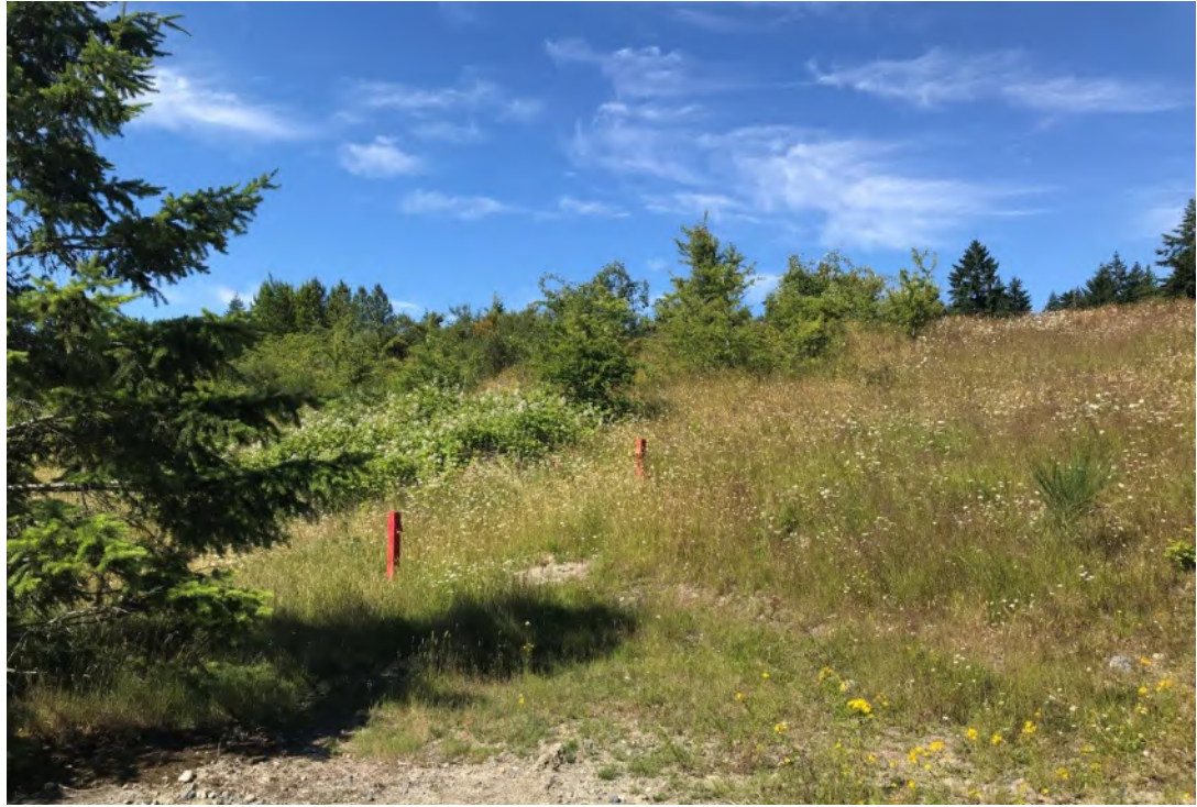
Photograph 3: Excavation 1a, facing southwest.
