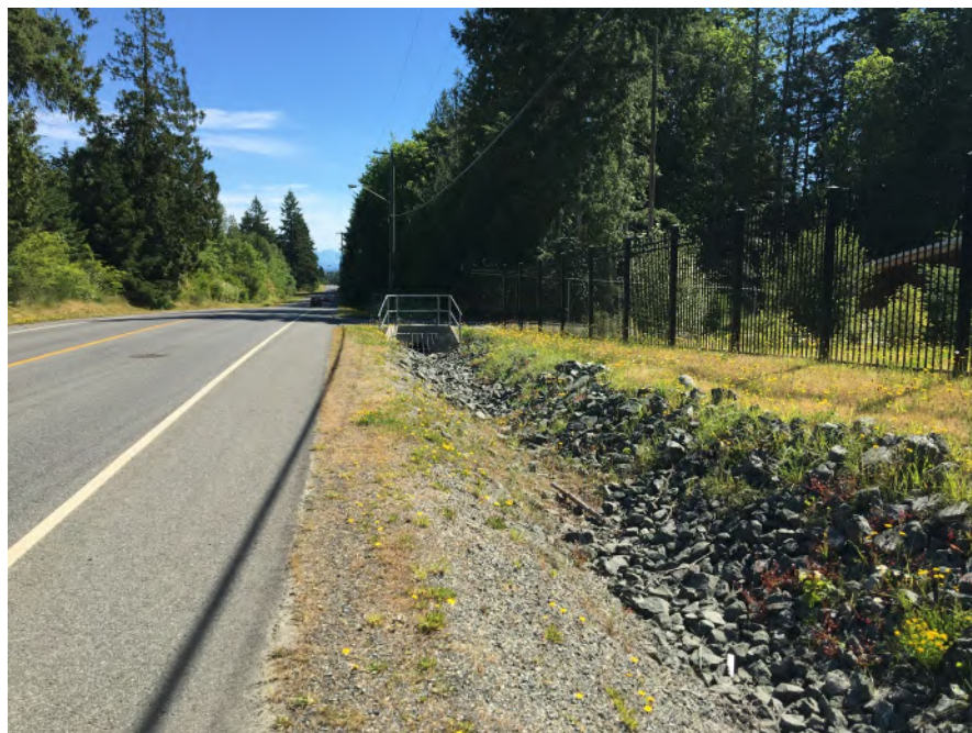
Photograph 2: Paved road and riprap ditch.
