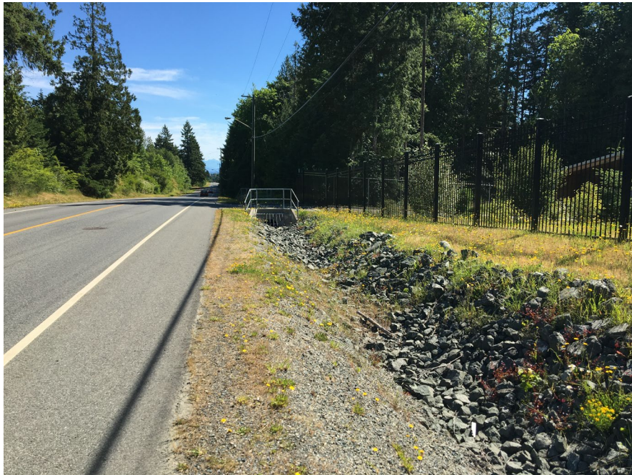
Photograph 2: Paved road and riprap ditch.
