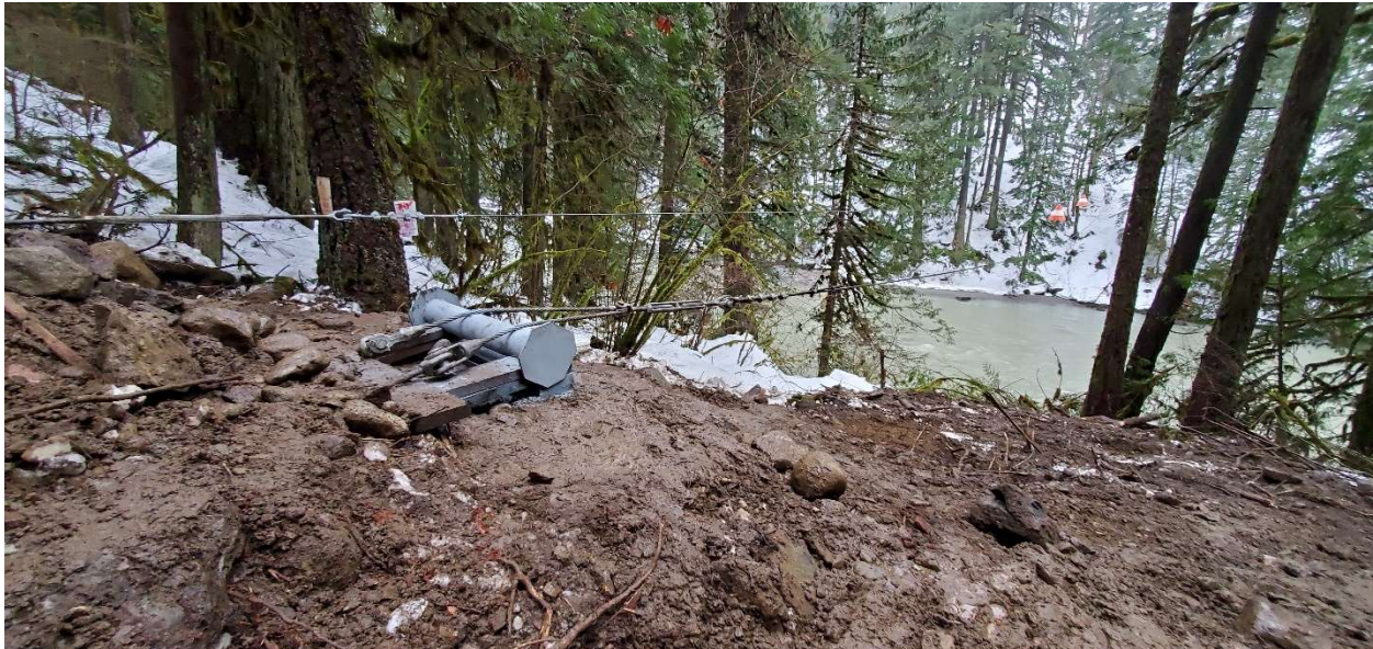
Figure 4: Example of Pipe Support
