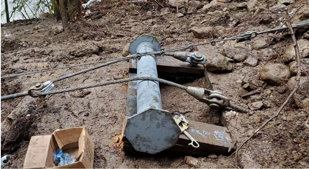
Figure 5: Pipe Support Example
