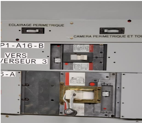
Picture 4 Circuit Breaker View – BAT A16 – 60A Perimeter Lighting
