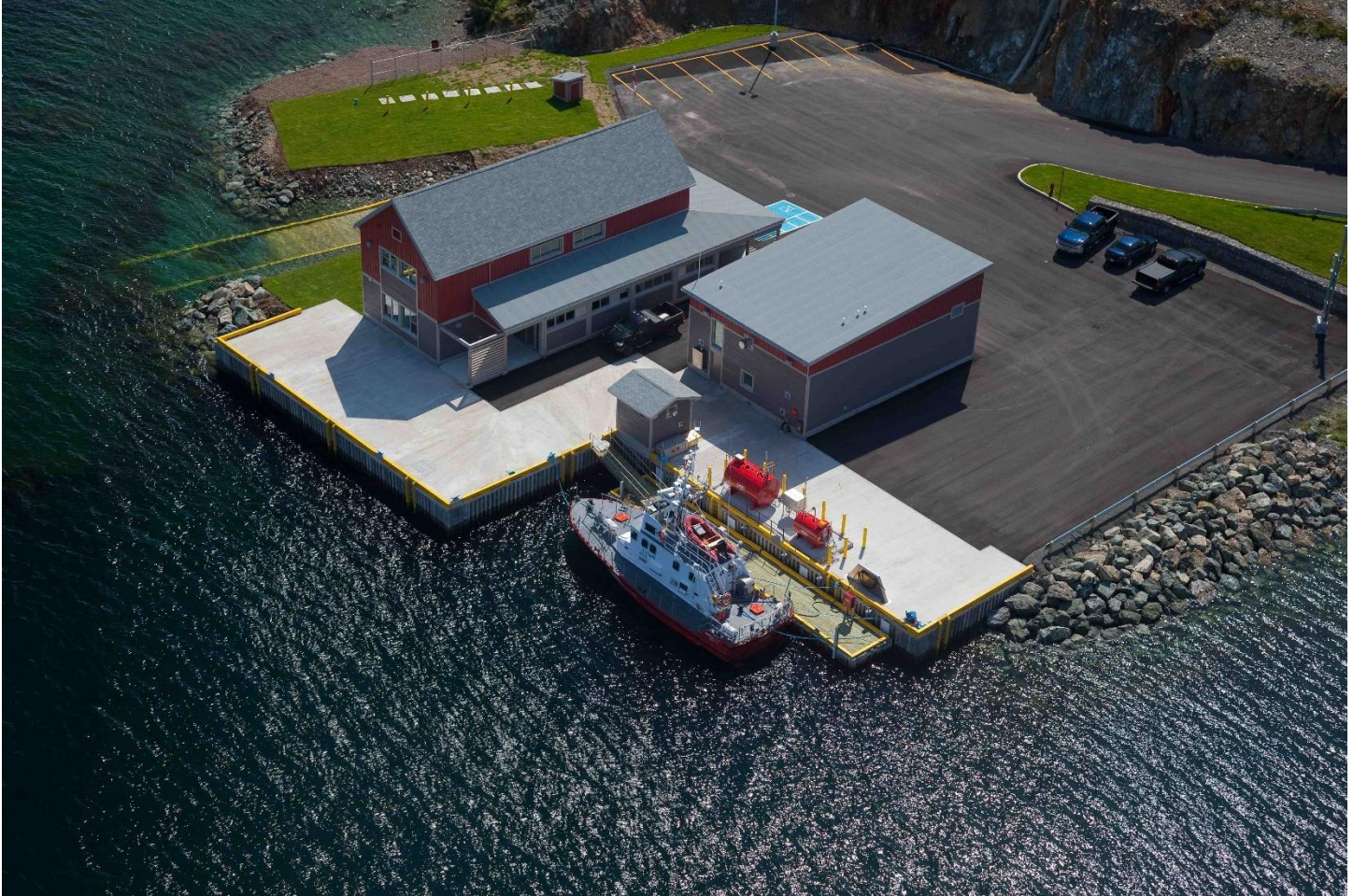
Figure 2 Site Photograph of Project Location in Burin, NL.
