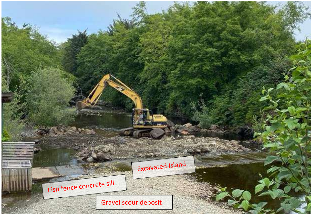
Figure 3: 2020 Outflow Channel Restoration Works – adapted from Instream Fisheries Research Inc. Report.
