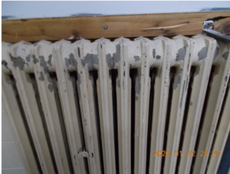
Photo 41: Light beige paint sampled from the radiator in the basement office 034, Location 38 contains 11100 ppm lead (DST 2020 Sample ID 040333-LP08).
