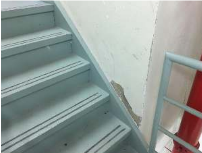
Photo 28: Textured cementitious wall parge in building stairwells was confirmed by laboratory analysis to not contain asbestos.
