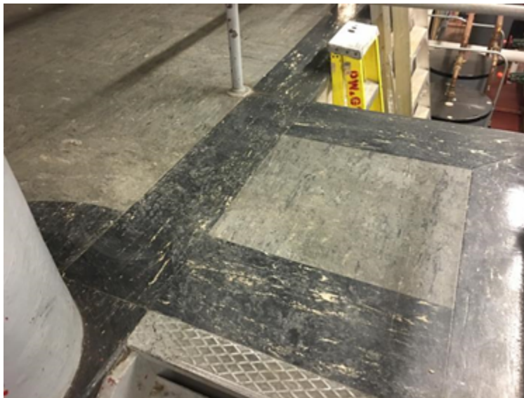
Photo 14: Mastic associated with vinyl floor materials in upper area of sub-basement mechanical room 003/entryway from basement level, contains regulated amounts of asbestos (Historical DST 2016 Sample ID 25657-series 39 & 40).
