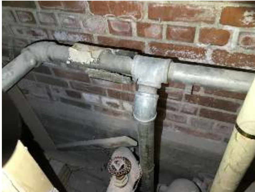
Photo 19: Poor condition asbestos-containing layered cardboard wrap pipe insulation in wall hatch, Ground Floor, Room 155 side washroom.
