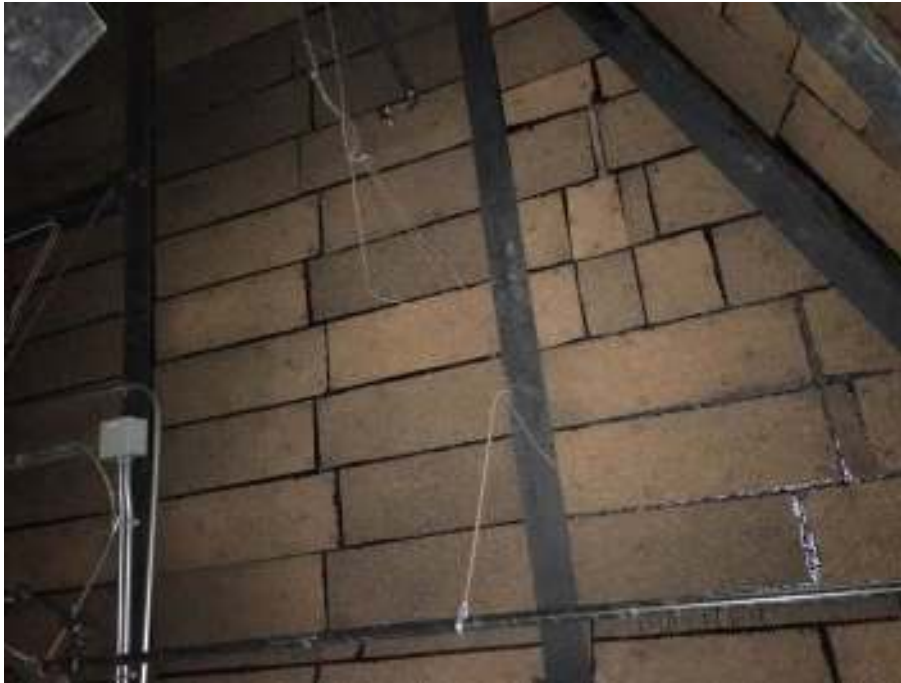
Photo 24: Tar and cork materials lining the interior roof structure above the 3 rd floor was confirmed by laboratory analysis to not contain asbestos.
