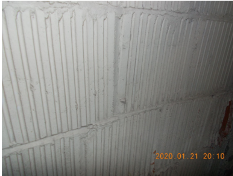
Photo 39: White wall paint sampled from the terracotta walls leading to the catacombs in the sub-basement, Location 1 contains 401 ppm lead (DST 2020 Sample ID 040333-LP01).
