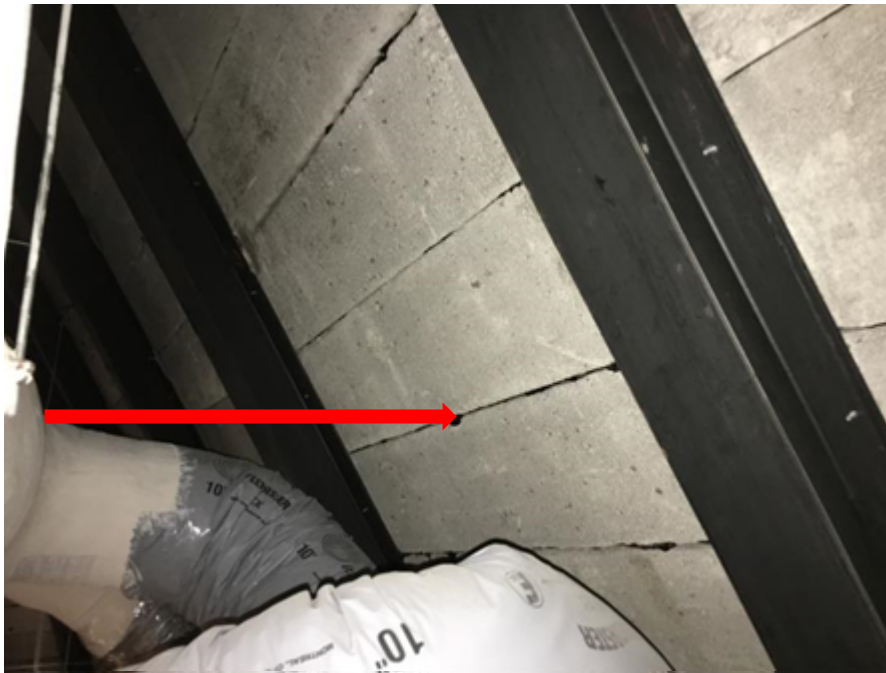
Photo 12: Tar, visible in joints of pre-cast cementitious panels that comprise the interior roof structure, 1 st Mechanical Floor, contains regulated amounts of asbestos. The cementitious panels themselves were confirmed by laboratory analysis to not contain asbestos ((Historical DST 2016 Sample ID 25657-series 18).
