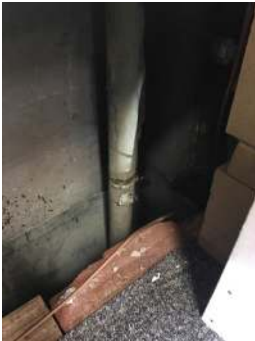
Photos 20 and 21: Poor condition asbestos containing insulation and debris, inside wall covering, basement, Room 082 (north wall).
