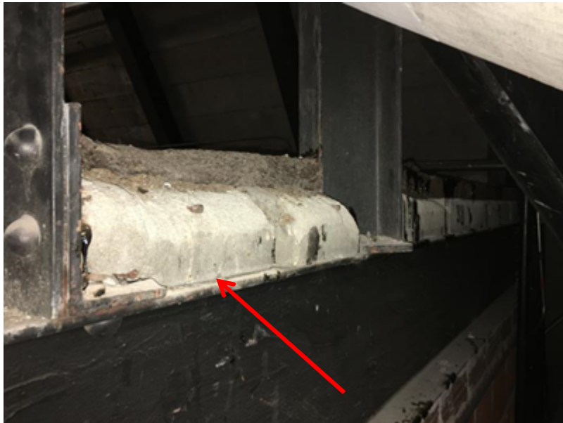
Photo 27: Cementitious floor fill beneath cork floors throughout the 1 st Mechanical Floor, was confirmed by laboratory analysis to not contain asbestos.
