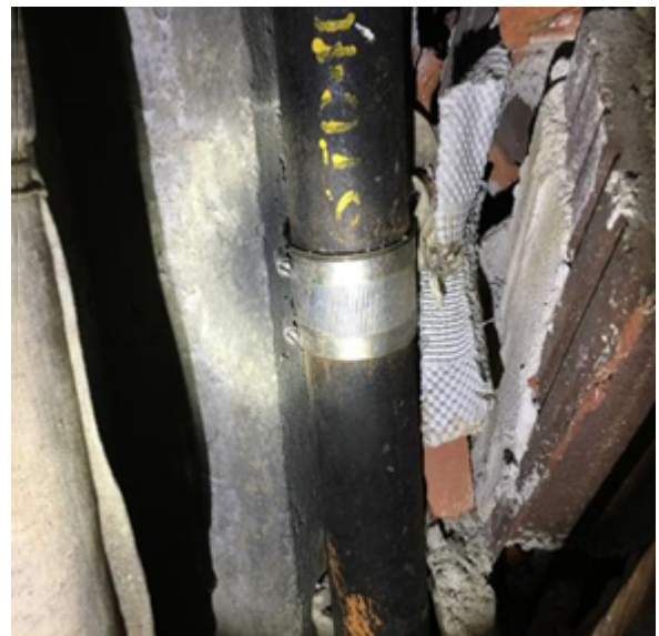
Photos 20 and 21: Poor condition asbestos containing insulation and debris, inside wall covering, basement, Room 082 (north wall).
