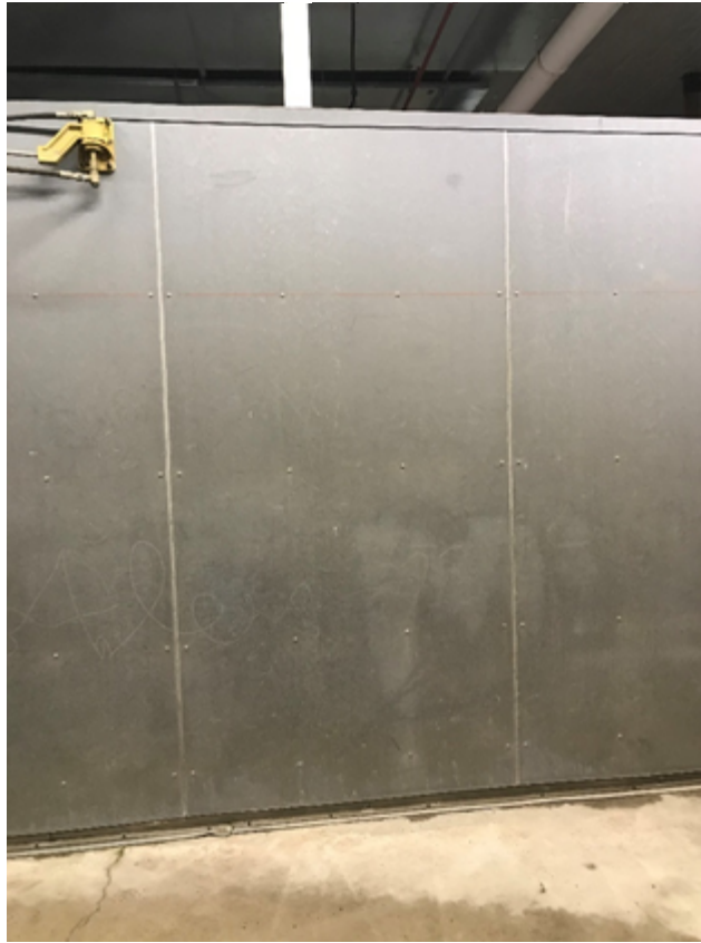
Photo 37: Suspect Transite board identified in the wash bay of the parking garage is assumed to contain asbestos.
