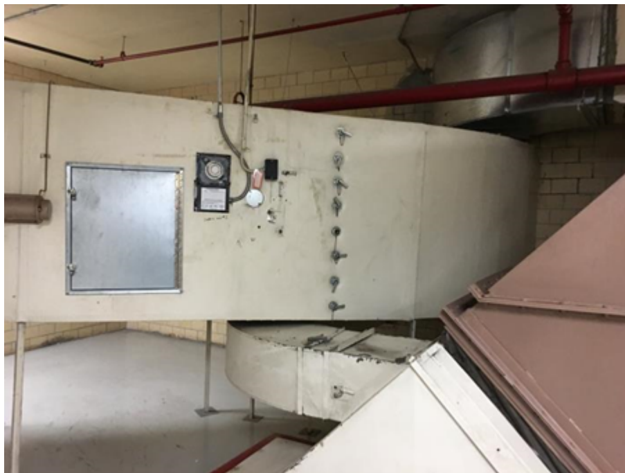
Photo 23: Parging over fiberglass duct insulation contains regulated amounts of asbestos (Room 0039, Sub-basement pictured above).
