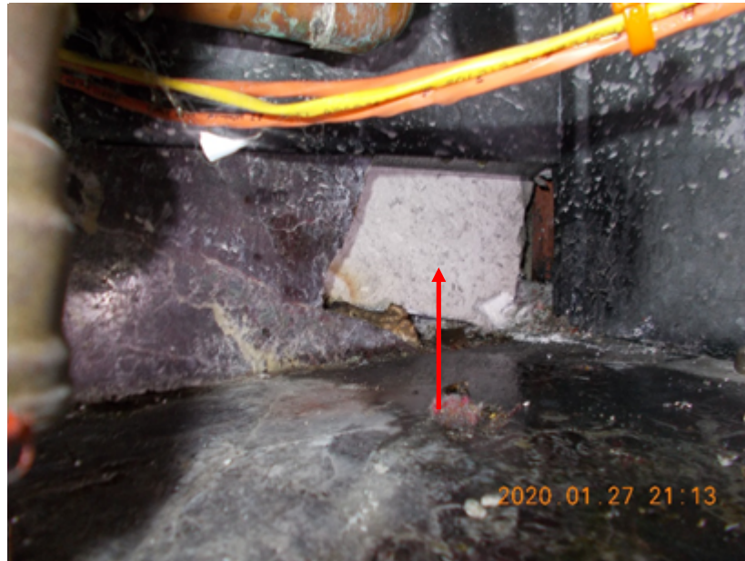
Photo 5: Friable when disturbed white fibrous insulation associated with radiators throughout the building was confirmed to contain 15% Amosite asbestos (DST 2020 Sample ID 040333-series 92).
