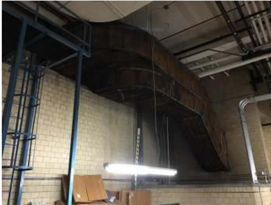
Photo 22: Duct insulation, Room 008, Sub-basement, contains regulated amounts of asbestos.
