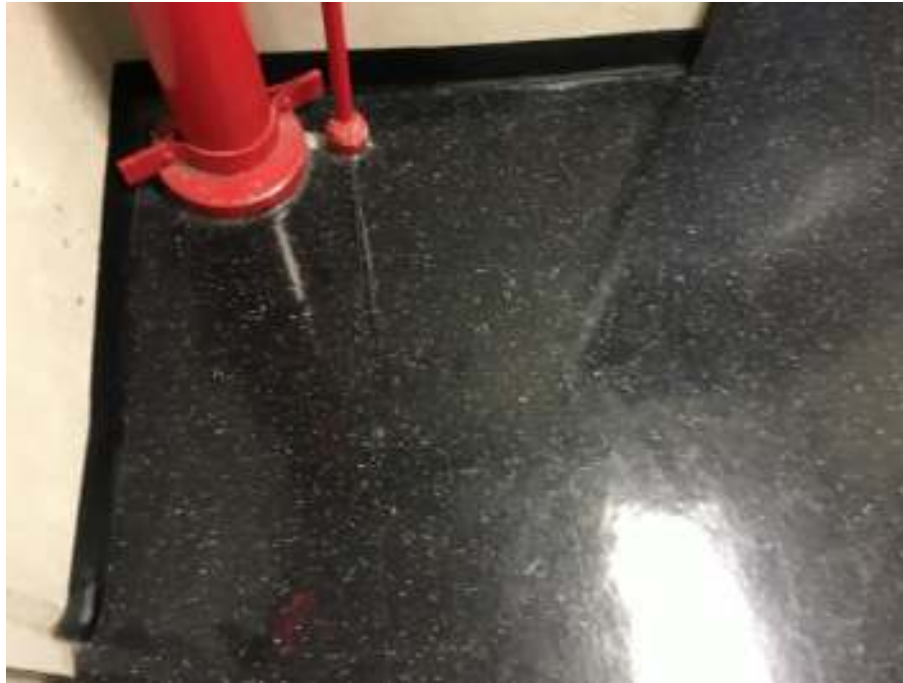
Photo 31: 12"x12" Vinyl floor tiles, black with white dots observed in select elevator lobbies, and stack 1 and 2 library areas was confirmed to not contain asbestos.
