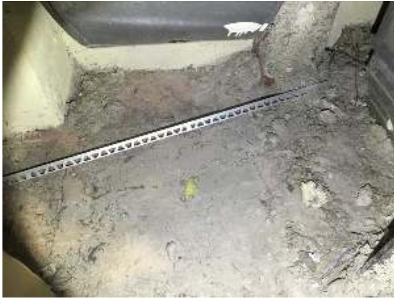
Photo 26: 3 rd Floor fill and textured cementitious coat on column were confirmed by laboratory analysis to not contain asbestos.
