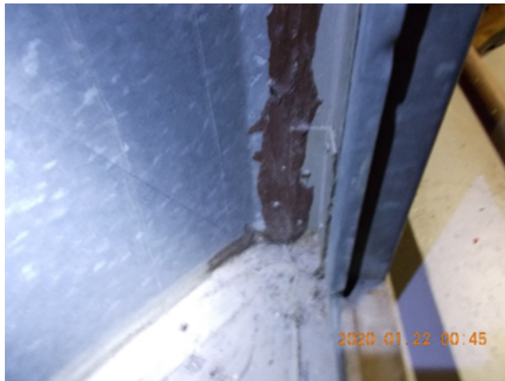
Photo 2: Non-Friable brown duct mastic sampled from inside AHU Unit #11 in the sub basement room 0010, Location 16 was confirmed to contain 2% Chrysotile asbestos (DST 2020 Sample ID 040333-series 71).
