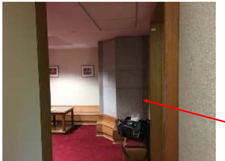
Photo 10: Mortar associated with stone panels in 3 rd Floor sitting area was confirmed to contain 1% Chrysotile asbestos (Historical DST 2016 Sample ID 25657-series 02).
