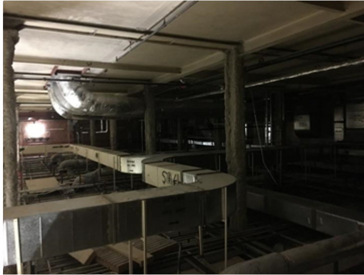
Photo 11: Cementitious parging throughout the ceiling of the mechanical area above the 3 rd Floor Library (south) contains 1% Chrysotile asbestos (Historical DST 2016 Sample ID 25657-series 16).
