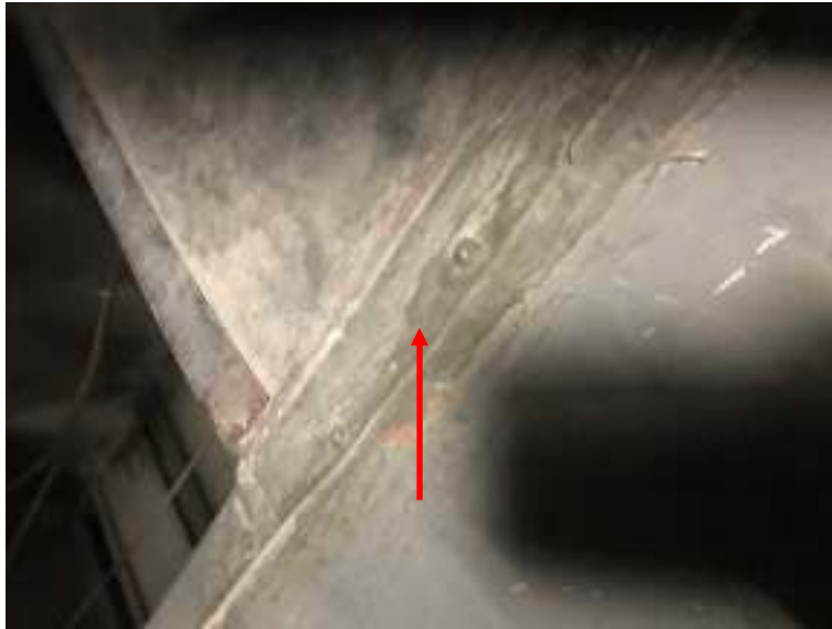
Photo 3: Non-Friable grey/brown caulking/mastic sampled from inside AHU Unit #1, 2 and 4 in the sub basement room 003 (central mechanical room), Location 10 was confirmed to contain 2% Chrysotile asbestos (DST 2020 Sample ID 040333-series 78).
