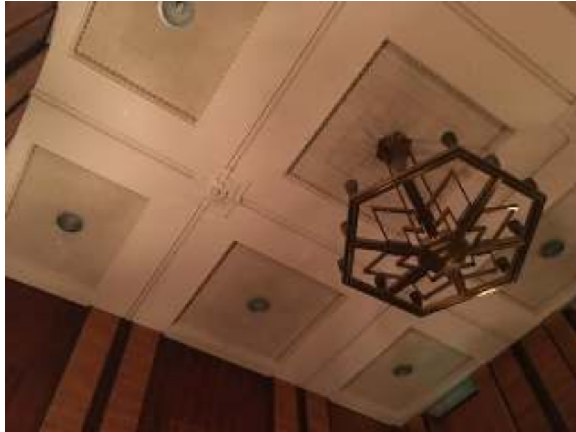
Photo 33: 1'x1' Ceiling tiles, typical of East and West Federal Court Chambers, Ground Floor, are suspected to contain asbestos.
