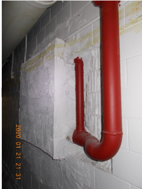
Photo 1: Friable (when disturbed) rough parge patch, observed in the sub basement room 0020 Northeast corridor, Location 8, sampled and confirmed to contain 1% Tremolite asbestos (DST 2020 Sample ID 040333-series 66).
