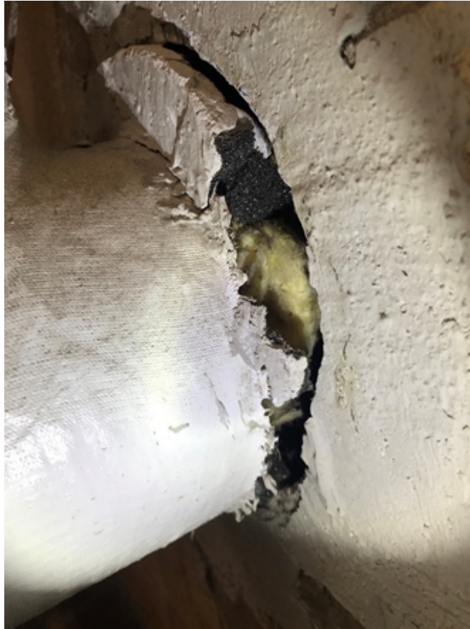
Photo 43: Foamglass observed at a pipe penetration in the central mechanical room 0017 in the sub-basement (near the door to the steam tunnels).
