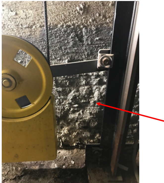
Photo 9: Friable when disturbed thin parging/rough coat associated with the Judges elevator shaft walls, Location C was confirmed to contain 1% Chrysotile asbestos (DST 2020, Sample 40333-series 146);
