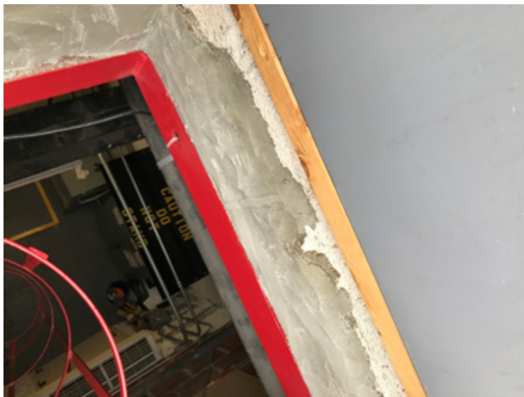
Photo 8: Friable when disturbed thin grey parging associated with the rooftop hatches above room 342 and 345 (elevator mechanical rooms) was confirmed to contain 1% Chrysotile asbestos (DST 2020 Sample ID 040333-series 142).
