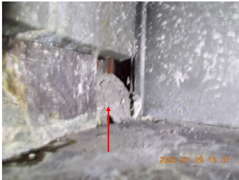
Photo 6: Friable when disturbed thin grey parging associated with radiators throughout the building was confirmed to contain 5% Amosite asbestos (DST 2020 Sample ID 040333-series 138).
