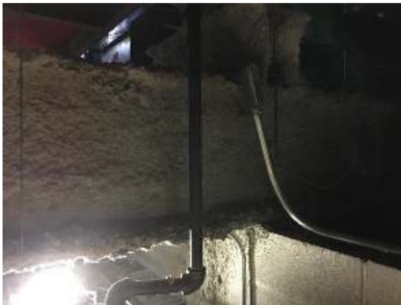
Photo 25: Spray fireproofing on beams and columns of the 3 rd Floor and above was confirmed by laboratory analysis to not contain asbestos.
