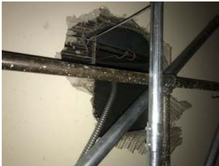
Photo 4: Friable when disturbed smooth over rough plaster walls and ceilings sampled throughout the building was confirmed to contain 0.5-1% Chrysotile asbestos (DST 2020 Sample ID 040333-series 82, 99, 111, 139, and Historical DST 2016 Sample ID 25657 -series 04, 27, 33).
