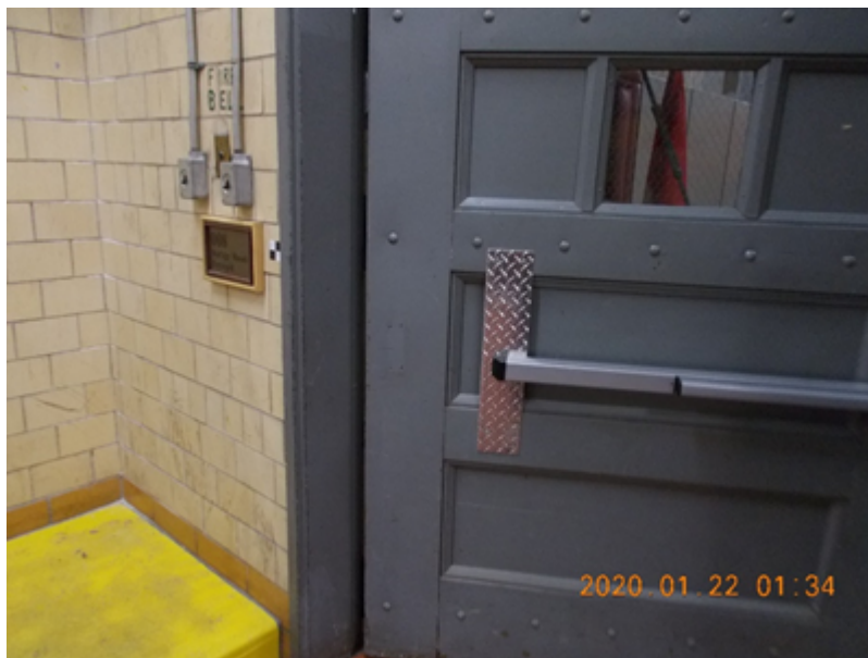
Photo 40: Dark grey paint sampled from the metals doors leading to room 008 in the sub-basement, Location 23 contains 4340 ppm lead (DST 2020 Sample ID 040333-LP07).
