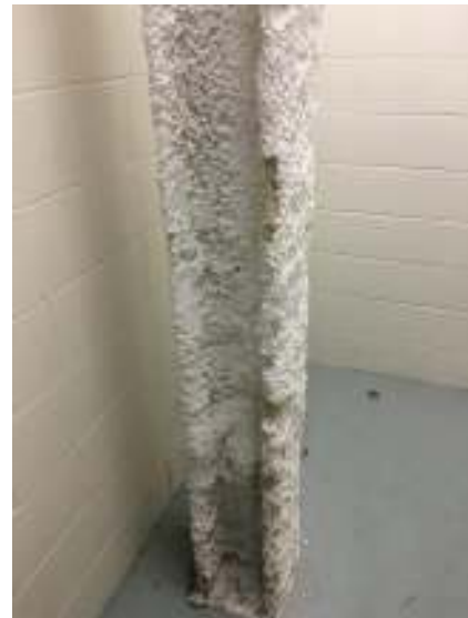
Photo 28: Textured cementitious wall parge in building stairwells was confirmed by laboratory analysis to not contain asbestos.
