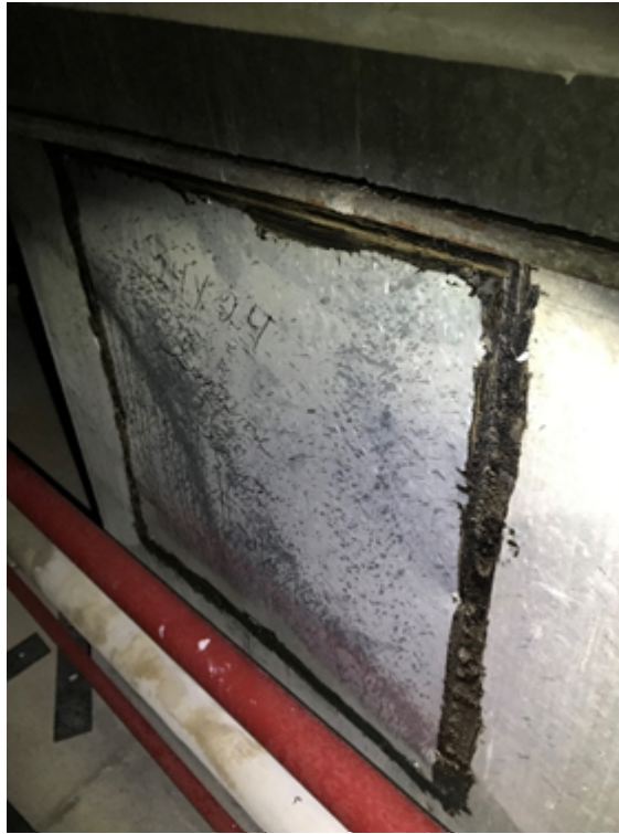
Photo 7: Non Friable tar caulking associated with duct hatch in the Mezzanine above room 0088 in the sub-basement, Location 263 was confirmed to contain 8% Chrysotile asbestos (DST 2020 Sample ID 040333-series 141).
