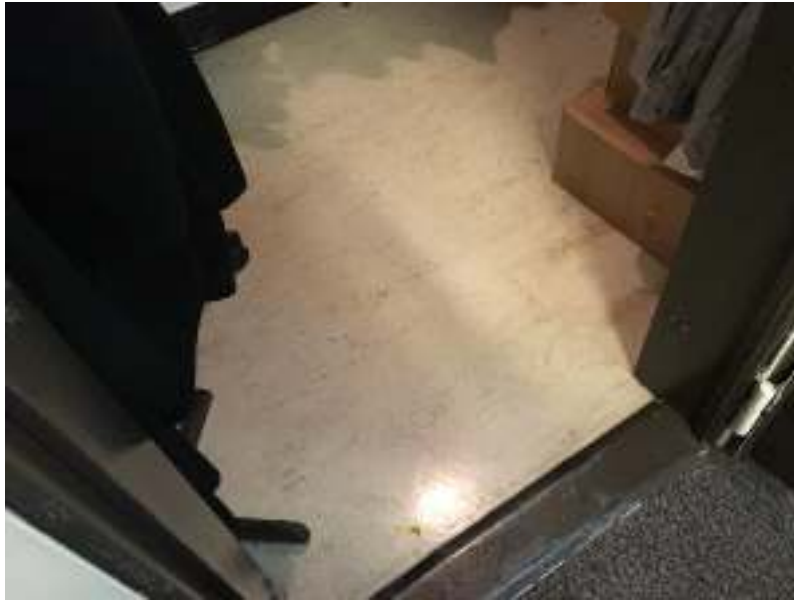
Photo 15: Vinyl floor tiles and associated mastic in the vault of Room 086, Basement, contains regulated amounts of asbestos(Historical DST 2016 Sample ID 25657-series 48).
