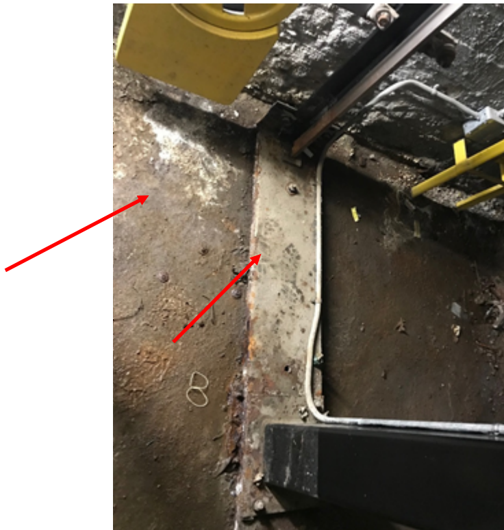
Photo 42: Grey paint sampled from the Judges elevator pit floor and the steel beam within the pit was confirmed to contain 2050 and 3480 ppm lead (DST 2020 Sample ID 040333-LP17 & LP18).
