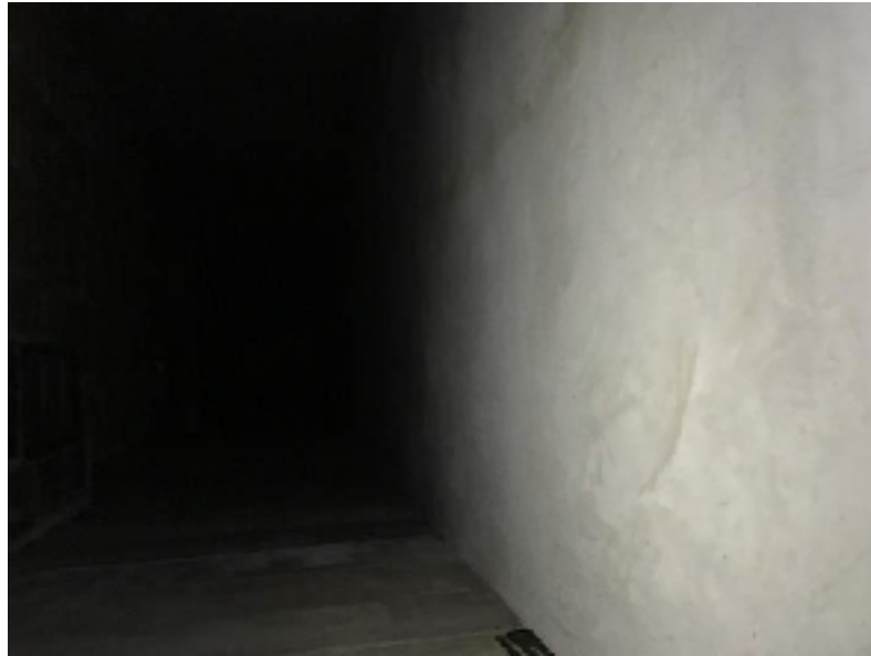
Photo 17: Wall parging (grey cement compound) in the catacombs (north) contains regulated amounts of asbestos (Historical DST 2016 Sample ID 25657-series 49).
