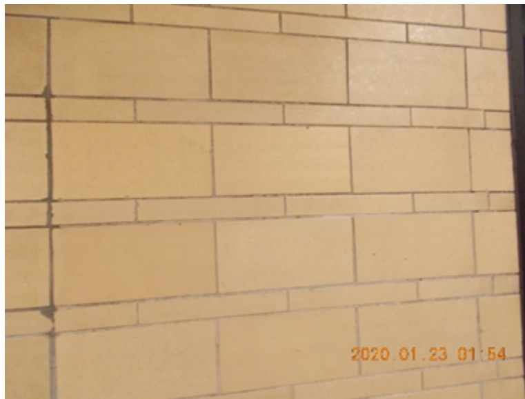
Photo 38: Mortar associated with tan glazed blocks (large and small) located in the basement north wall are confirmed to be non asbestos.
