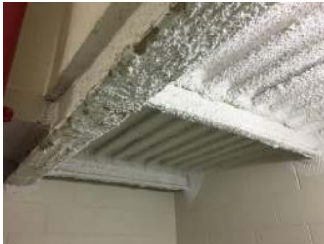
Photo 29 and 30: Spray fireproofing on bottom of northwest stairwell landing and throughout select areas of Second Mechanical Floor, was confirmed by laboratory analysis to not contain asbestos.
