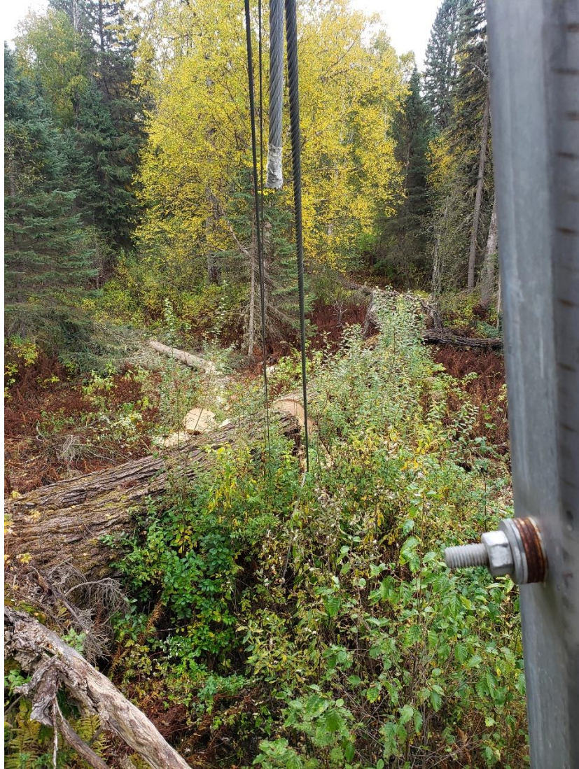
Figure 1: Fallen Tree on Right Bank Anchor Location
