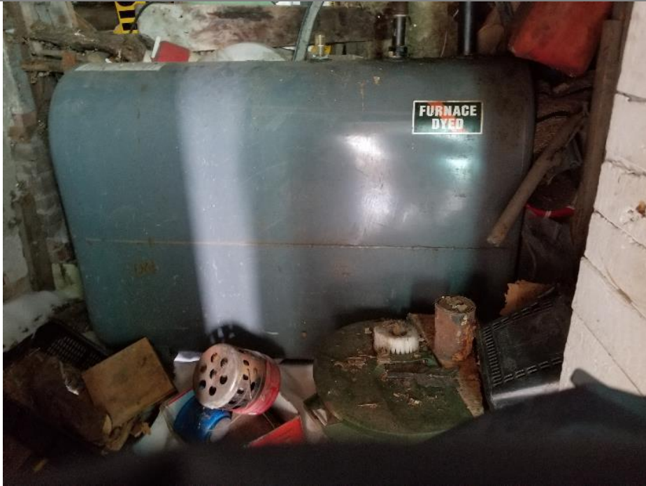
Photo 9: View of 909 L fuel oil above-ground storage tank on the second floor covered porch.
