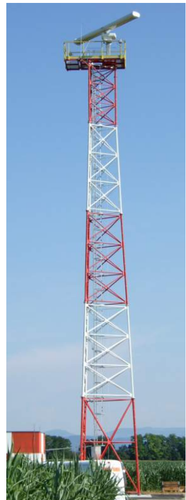
Figure 7.1 Three-legged lattice tower
