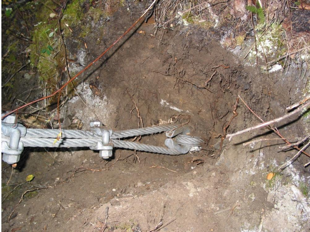
Photo 4. Unknown main cable anchor (right bank far side)
