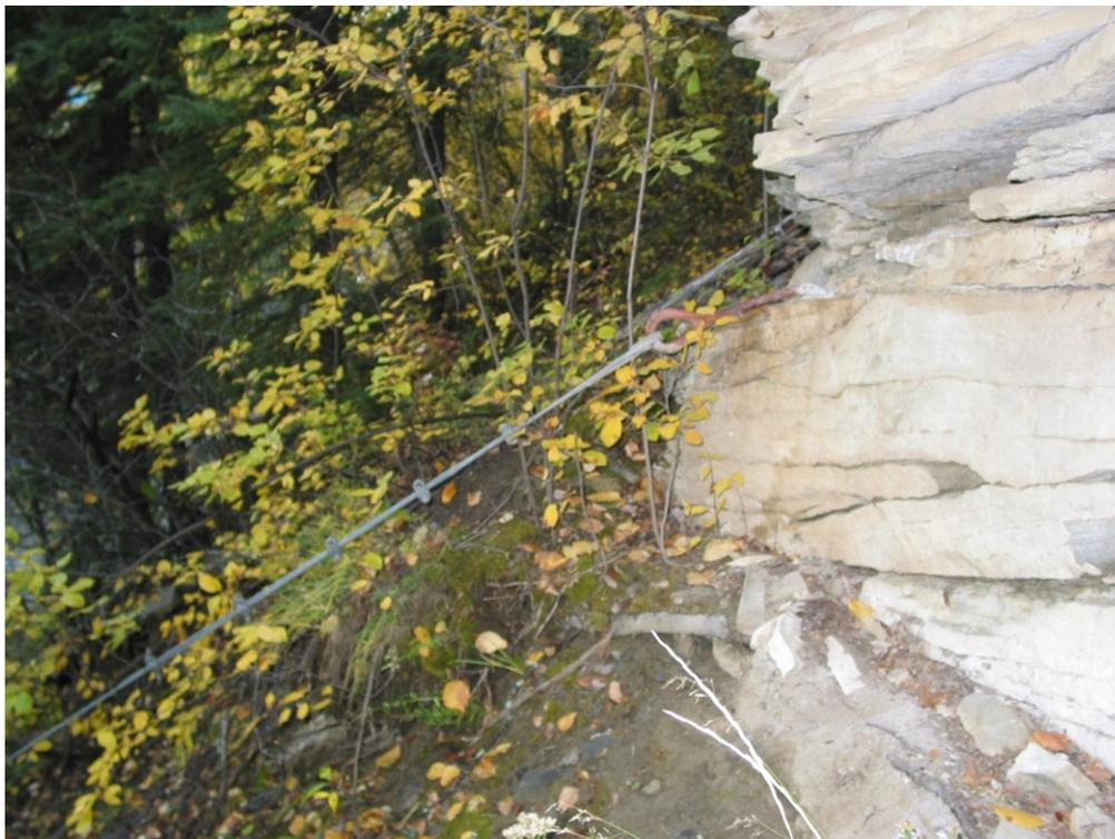
Photo 5. Marker cable anchor (right bank far side)
