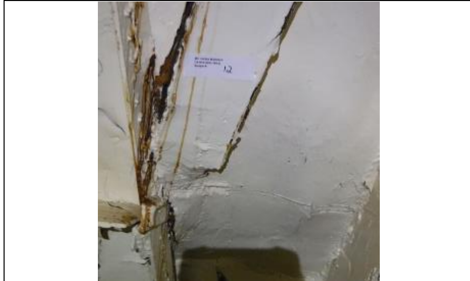
11. Cold store insulation – containing asbestos.
