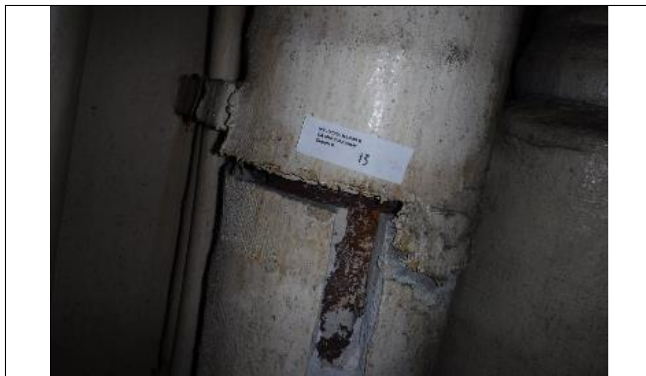
11. Cold store insulation – containing asbestos.
