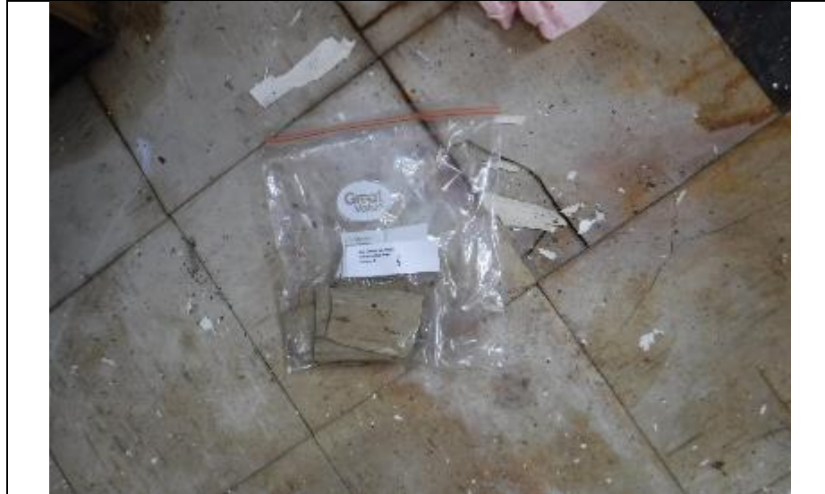
9. Floor tiles in wheelhouse and accommodation containing asbestos.
