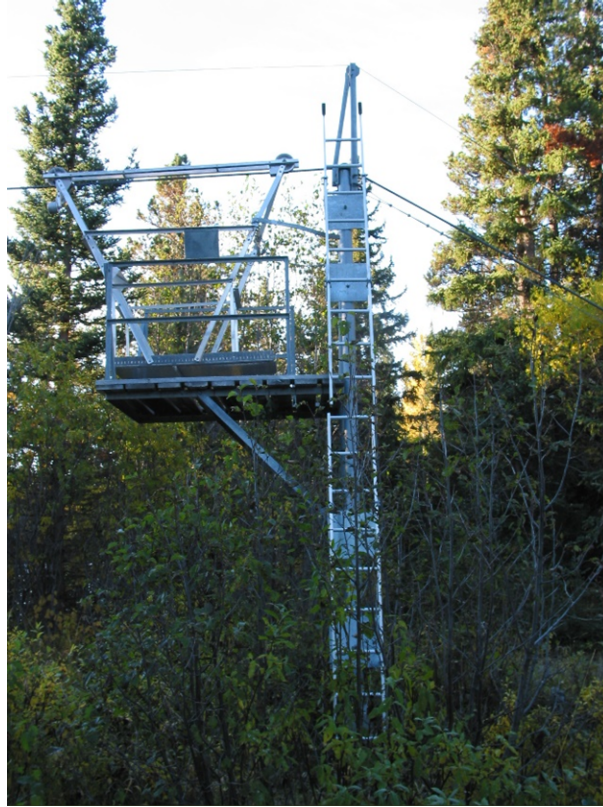
Photo 4. Left Bank Home-Side A-Frame (Side View)
