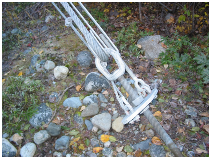
Photo 3. Right Bank Far-Side Anchor Connections
