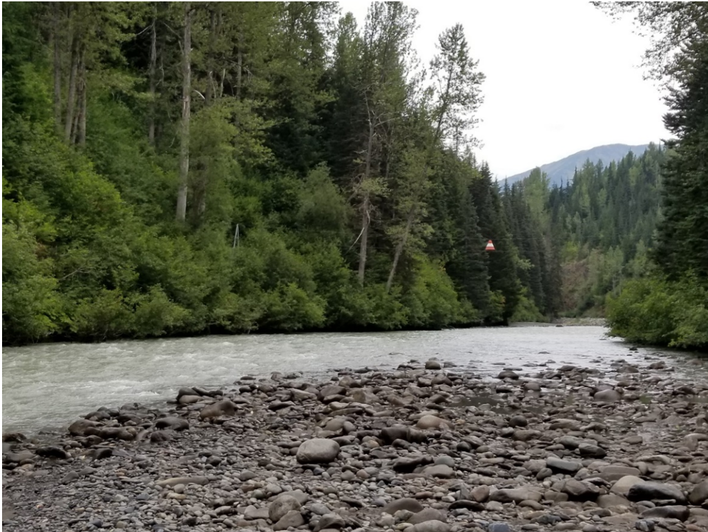
Photo 1. General View of Cableway
