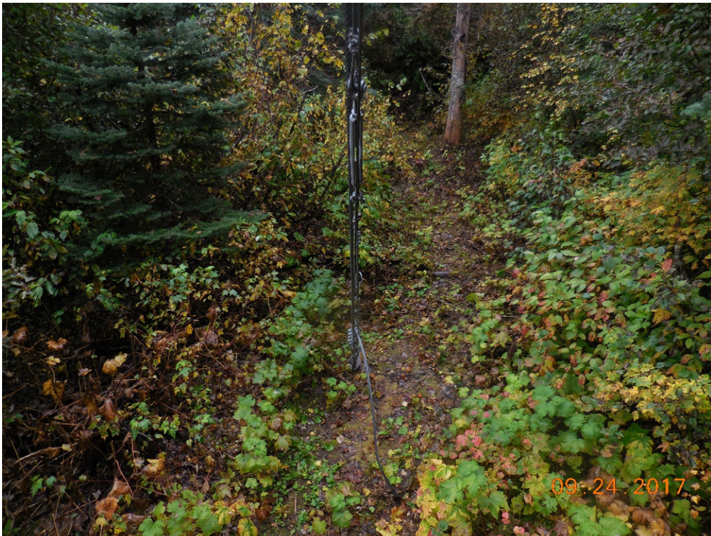
Photo 5. Far Side Anchor
