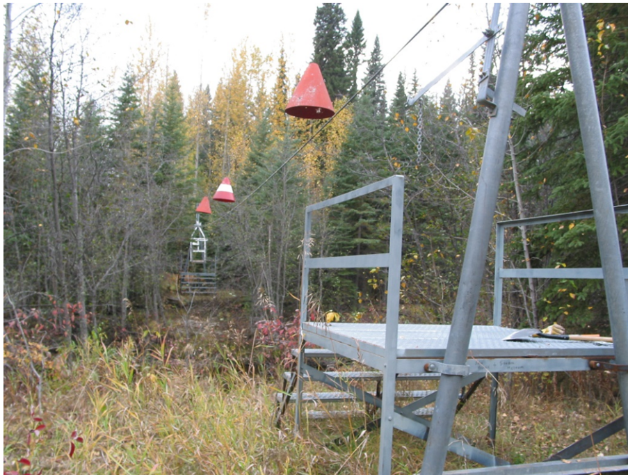
Photo 1. General View of Cableway
