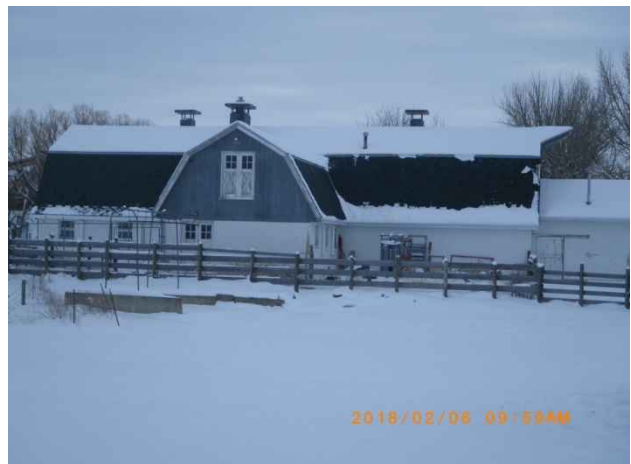
Photo 72. Exterior view of Large Barn (Building #102837), looking southeast-east.
