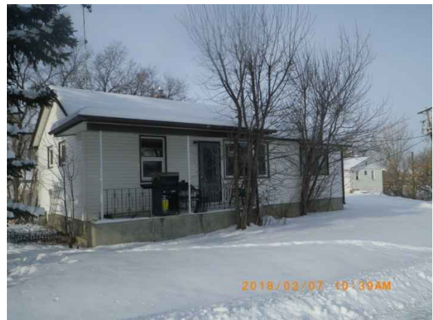
Photo 60. Exterior view of House AGR 280 (Building #102834), looking southwest.
