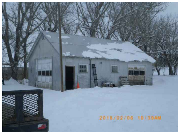
Photo 114. View of Metal Shop (Building #102836), looking northeast.
