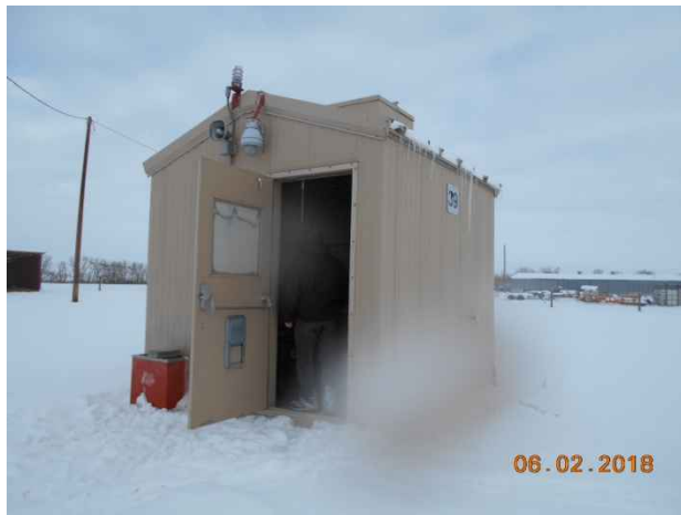
Photo 117. View of Pumphouse #2 (Building #102846), looking east-southeast.
