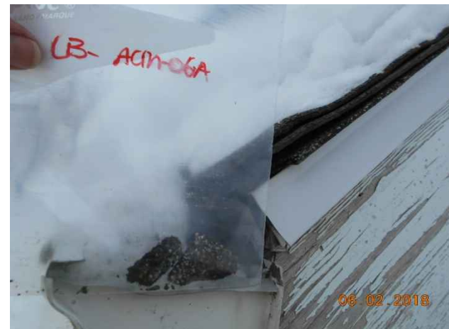
Photo 78. Sample locations LB-LB-ACM-06A to C; multicolour roof shingles (bottom layer).
