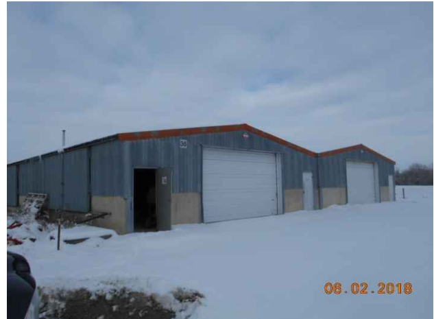
Photo 116. View of Feed and Machinery Shop (Building #102843), looking northwest.
