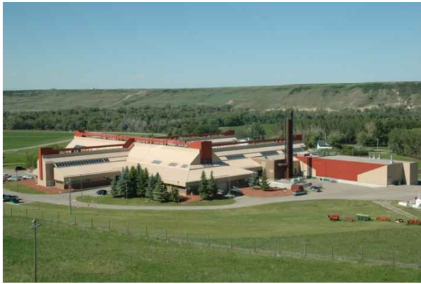
Photo 1. Overview of Main Lab (Building 014990).
