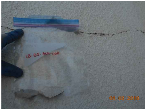
Photo 55. Sample location LB-B5-ACM-06A; exterior wall plaster.
