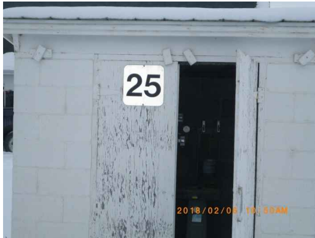
Photo 115. View of Scale House (Building #102841), looking southeast.
