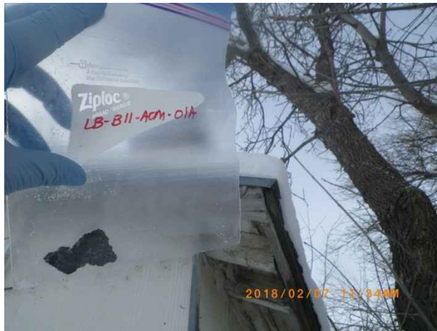
Photo 69. Sample locations LB-B11-ACM-01A to C; roof shingles.
