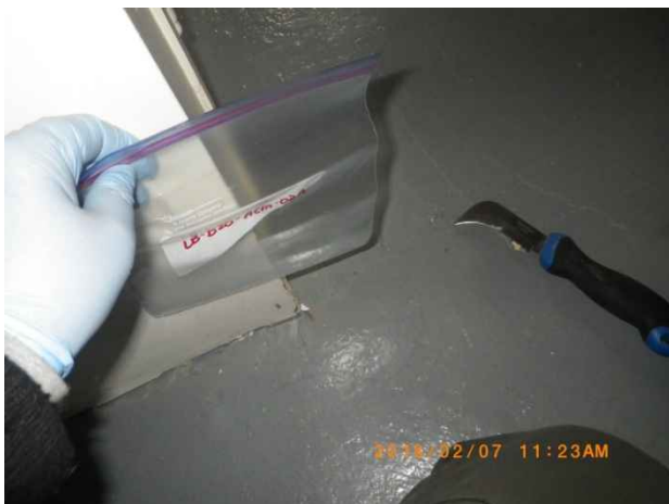
Photo 101. Sample location LB-B20-ACM-02A; drywall mud joint compound by basement bathroom.
