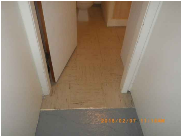
Photo 99. Tan 12"x12" floor tile in basement bathroom.
