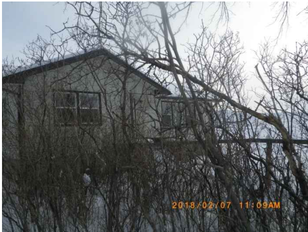
Photo 97. Exterior view of House AGR 284 (Building #102839), looking northwest.
