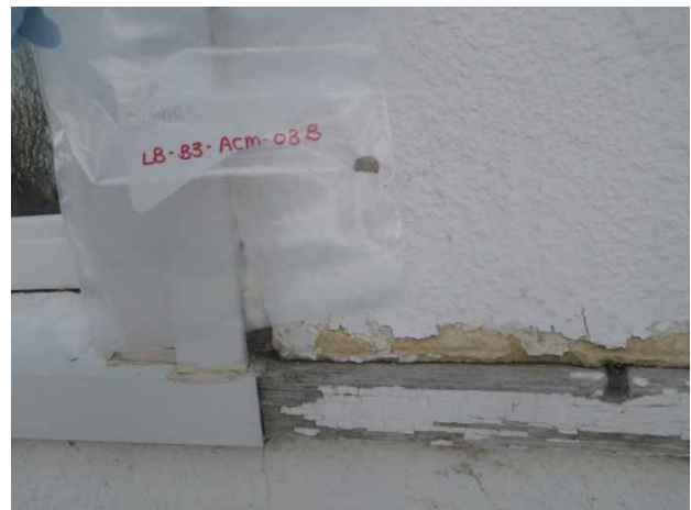
Photo 36. Sample location LB-B3-ACM-03B; exterior plaster (multi layers).
