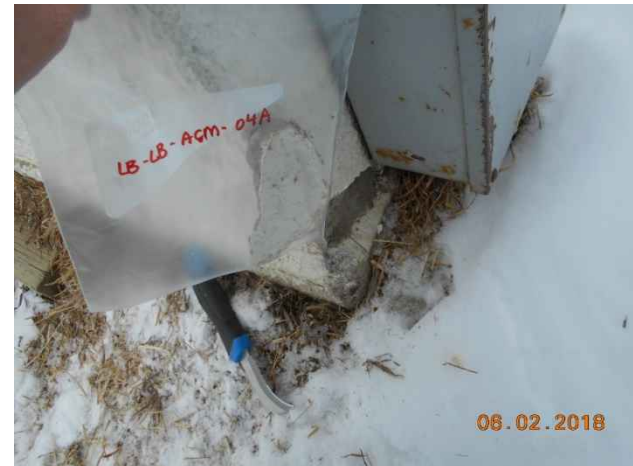
Photo 76. Sample locations LB-LB-ACM-04A to C; exterior wall plaster.
