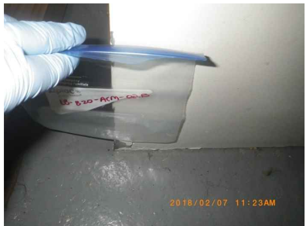
Photo 102. Sample location LB-B20-ACM-02B; drywall mud joint compound by basement bathroom.
