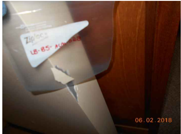
Photo 50. Sample location LB-B5-ACM-02B; dry wall/mud joint compound in front entry closet.
