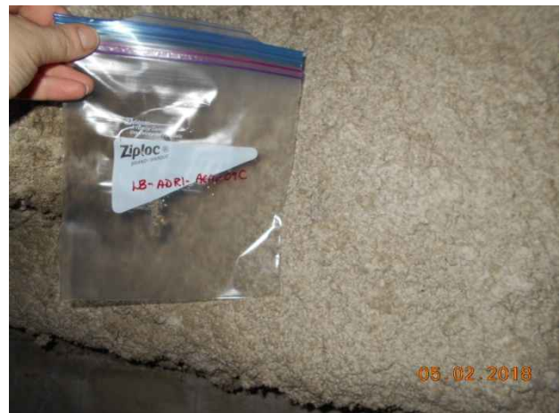
Photo 18. Sample location LB-ADRI-ACM-09C; spray on foam insulation in 400 Wing Crawlpace.
