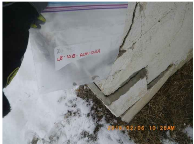
Photo 112. Sample locations LB-ISB-ACM-02A to C; exterior wall plaster.
