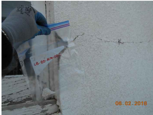
Photo 57. Sample location LB-B5-ACM-06C; exterior wall plaster.
