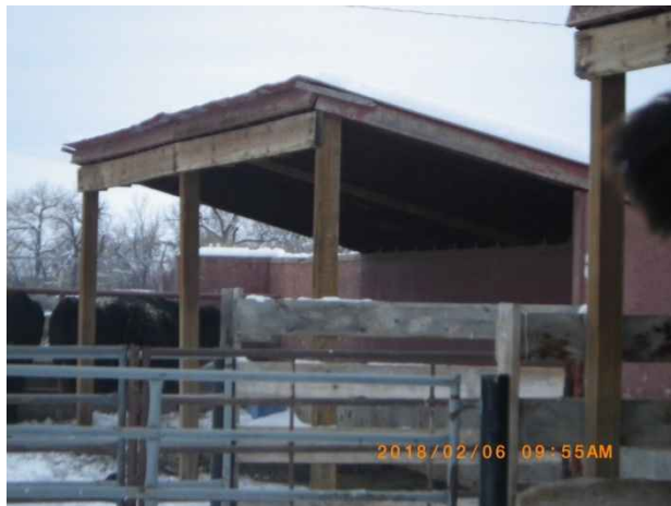
Photo 119. View of Lower Pens #1-8 (Buildings 102850-102856), looking southeast.
