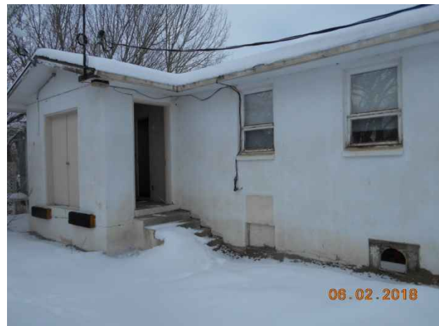
Photo 46. Exterior view of Student Residence (Building #102832), looking northwest.
