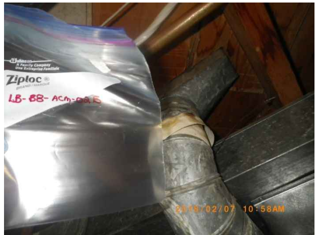
Photo 66. Sample location LB-B8-ACM-02B; paper-wrap around ducting (not sampled based on confirmed asbestos in sample LB-B8-ACM-02A).
