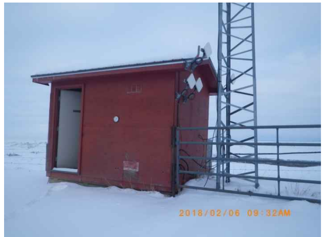
Photo 124. View of Radio Repeater Shack (Building #102867), looking southeast.
