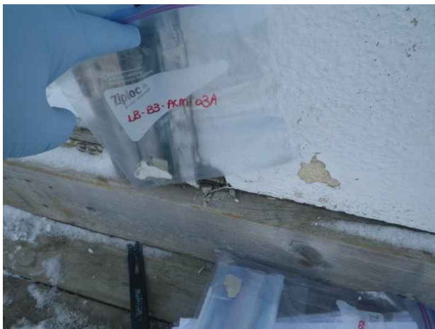
Photo 35. Sample location LB-B3-ACM-03A; exterior plaster (multi layers).
