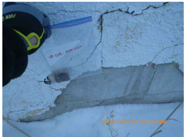
Photo 108. Sample location LB-CS3-ACM-02C (mis-labeled in image); exterior plaster (multiple layers).
