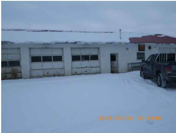
Photo 109. Exterior view of Dry Storage (Building #137925), looking northwest.
