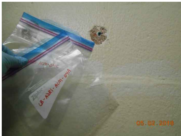
Photo 11. Sample locations LB-ADRI-ACM-04A to C; plaster coat on brick in R.418.
