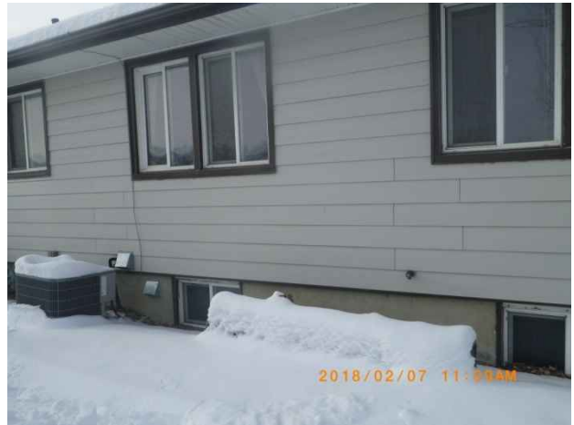
Photo 98. Exterior side view of House AGR 284.
