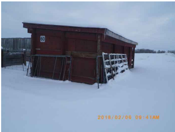
Photo 123. View of Isolation Sheep Shelter (Building #102866), looking northeast.
