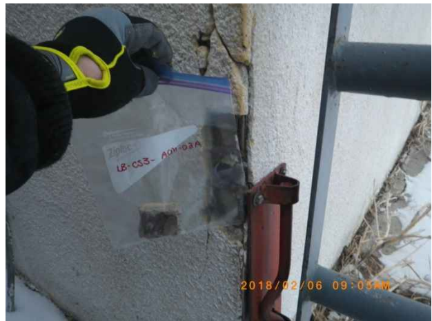
Photo 106. Sample location LB-CS3-ACM-02A; exterior plaster (multiple layers).
