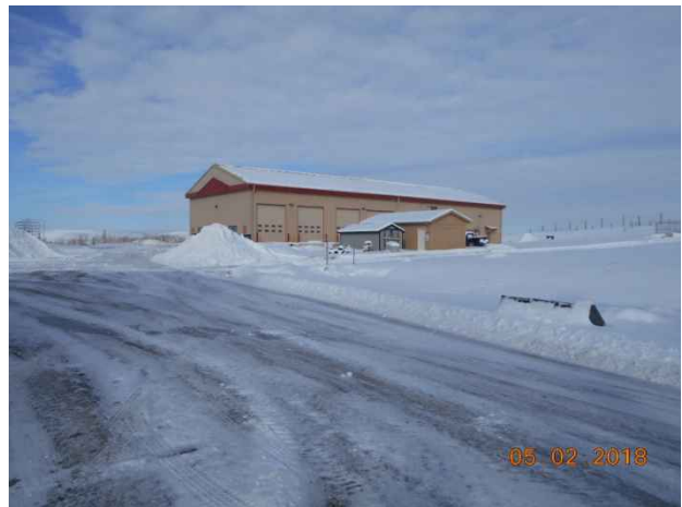
Photo 20. View of General Services Building (102829), looking northwest.
