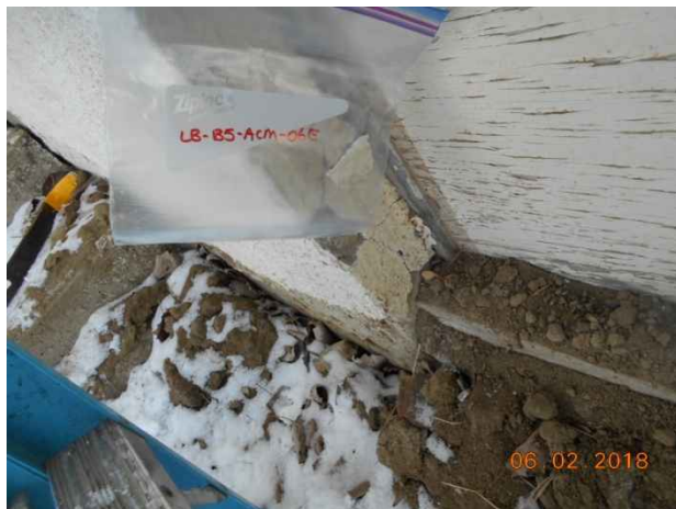
Photo 59. Sample location LB-B5-ACM-06E; exterior wall plaster.
