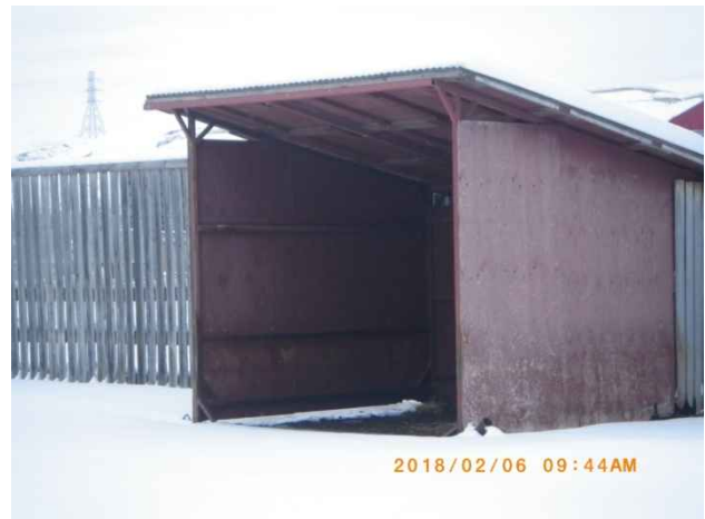
Photo 118. View of Lower Pens #1-8 (Buildings 102850-102856), looking southeast.
