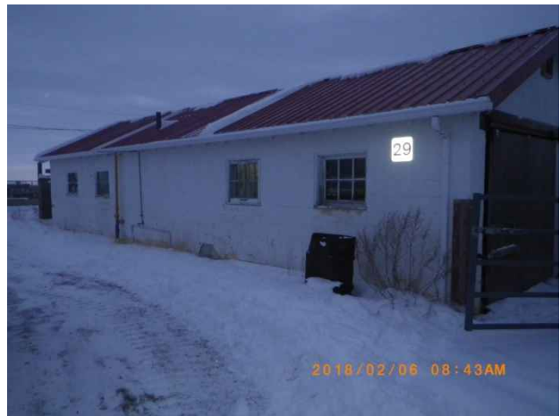
Photo 104. Exterior view of Isolation Sheep Barn (Building #102842), looking south.
