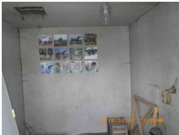
Photo 71. Sample locations LB-B11-ACM-03A to C; interior cement/transite board. Confirmed asbestos-containing materials (25% Chrysotile).
