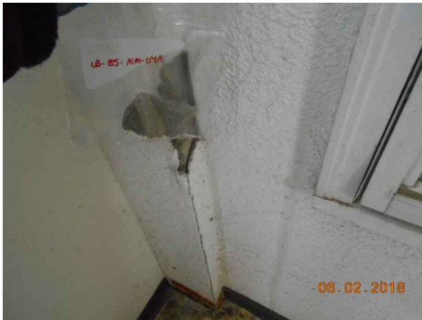
Photo 53. Sample locations LB-B5-ACM-04A to C; wall plaster on basement wall.
