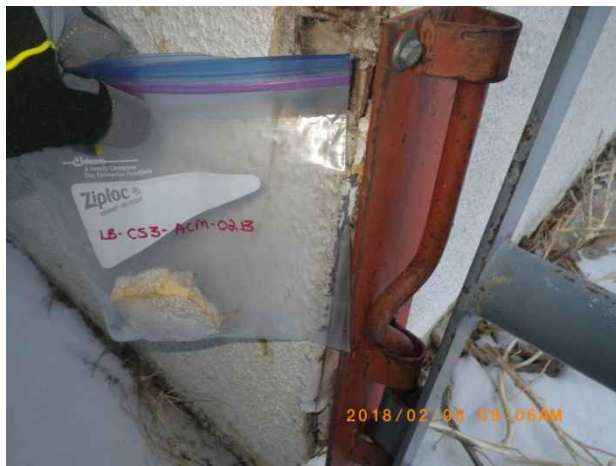
Photo 107. Sample location LB-CS3-ACM-02B; exterior plaster (multiple layers).
