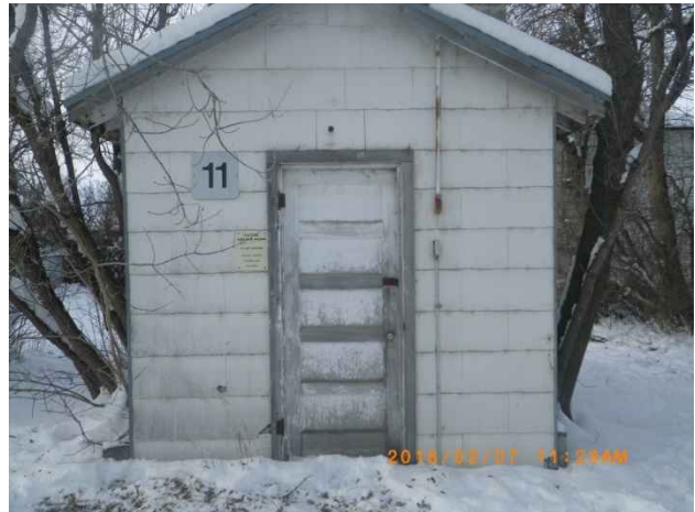
Photo 68. Exterior view of Pumphouse #1 (Building #102834), looking northeast.
