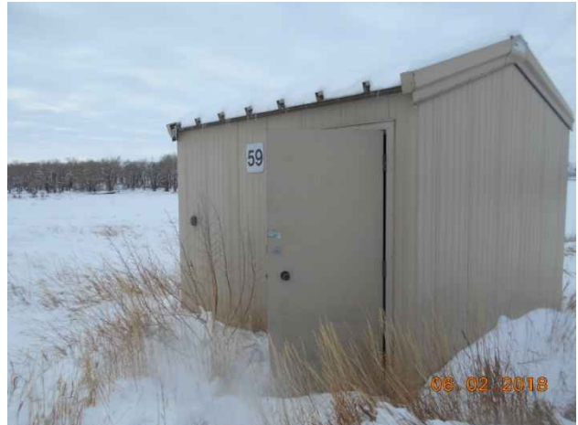
Photo 122. View of Pump House #3 (Building #102865), looking northeast.
