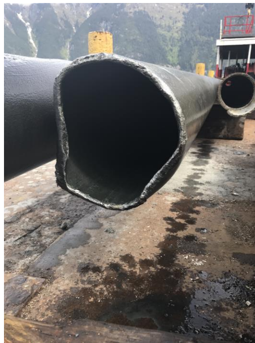
Photograph 1. Tip Damage from Driven Piles
