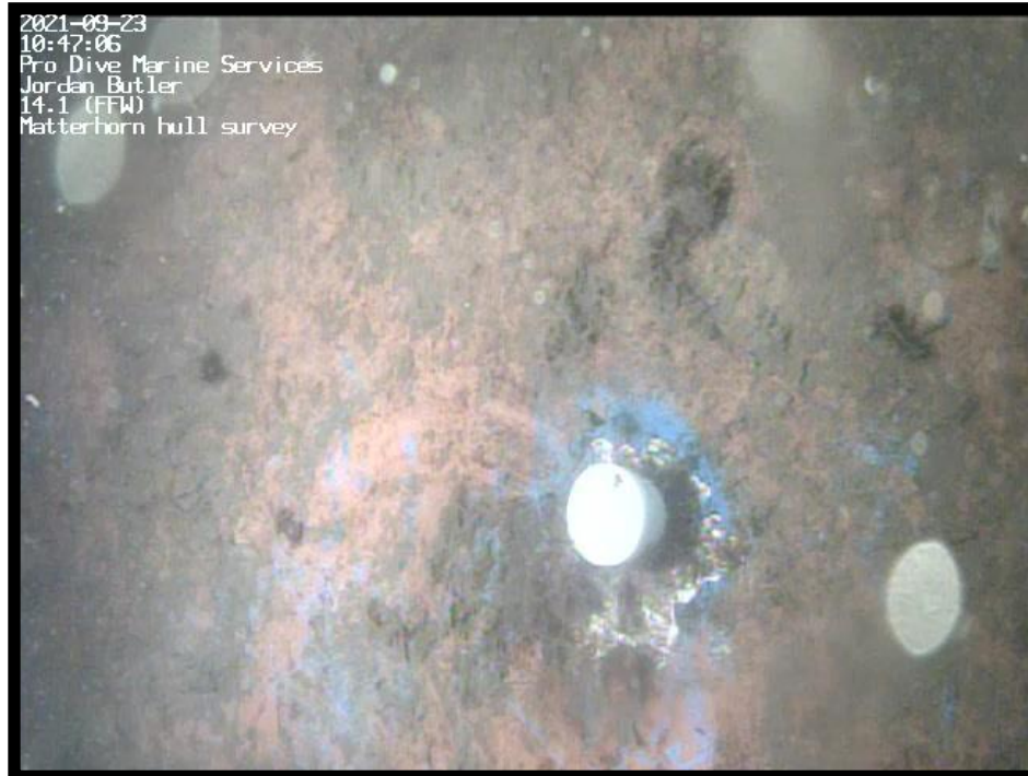
Figure 17 - Plug installed on starboard side.
