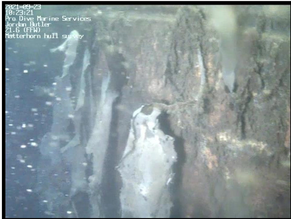
Figure 16 - Marine growth on keel near the stern area.
