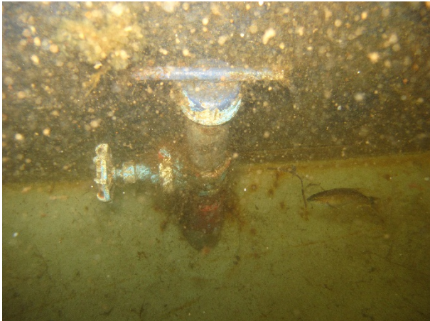
Shows pipe with cap installed.
