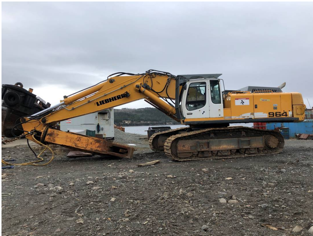
10. Excavator rigged with metal shears
