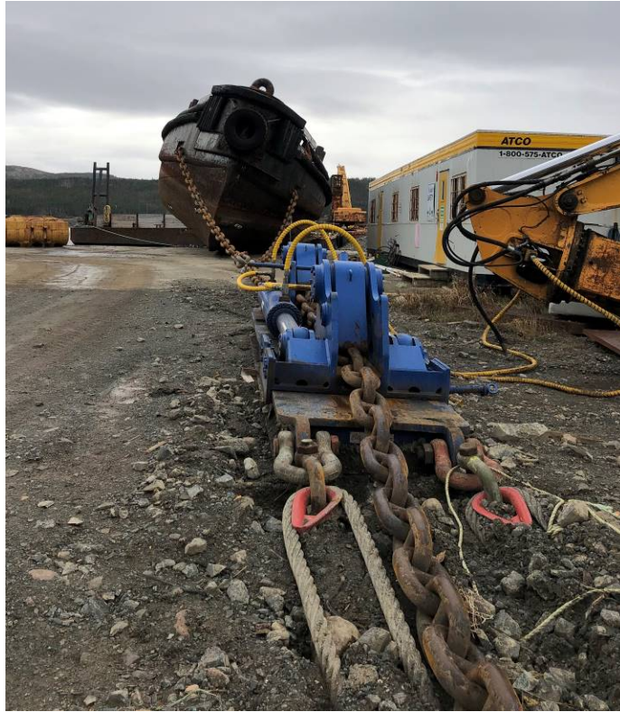
9. Remains of tug ex NORTHERN TUGGER connected to the chain puller
