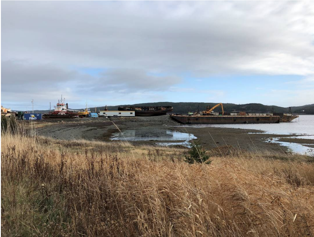
3. View facility looking north. MATTERHORN sunk behind the two barges
