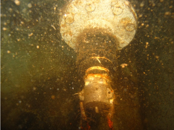
Shows pipe penetration capped with camlock cap.
