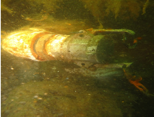
Shows penetration secured with end cap.
