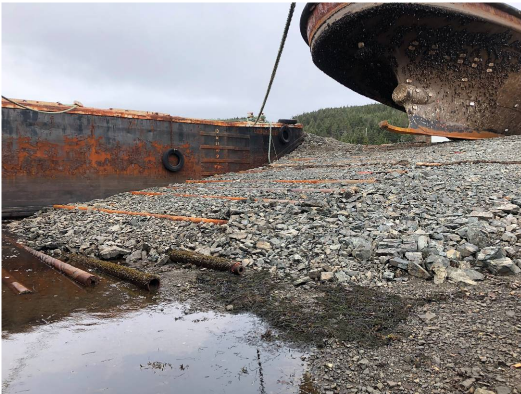
6. "Slipway" using drill pipe as skids
