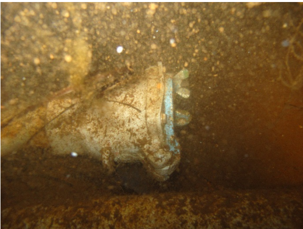
Shows vent secured with steel plate.
