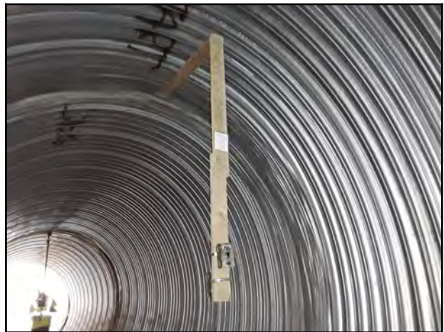
Photo 28 - Trail camera installed within the asset, at 21.00 m.
