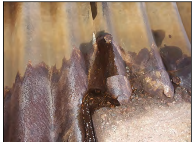
Photo 34 - V-4: Level 2 water infiltration at seam.
