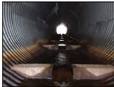
Photo 27 - Pipe has a total of 15 fish weirs installed.
