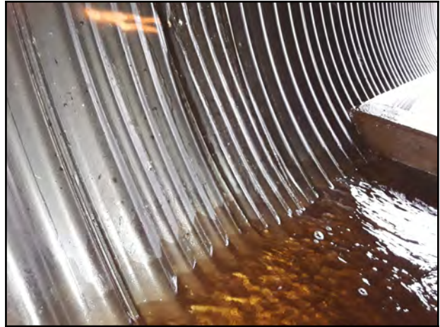
Photo 26 - V-1: Offset joint by approximately 40 mm with a visible coupler.
