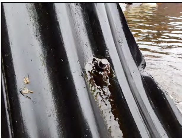
Photo 35 - V-7: Level 3 water infiltration at bolt with organic matter buildup.
