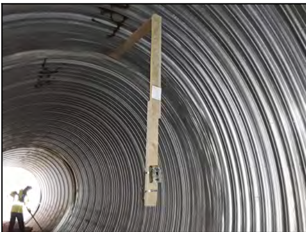
Photo 23 - V-2: Separated and offset joint by approximately 110 mm with visible filter fabric, and backfill material present.
