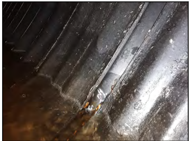
Photo 28 - V-3: Offset joint by approximately 30 mm with a visible coupler and level 3 water infiltration evident.
