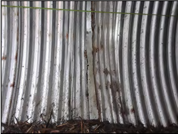
Photo 19 - V-1: Separated and offset joint by approximately 120 mm with visible backfill material, as well as surface corrosion at joint connection.
