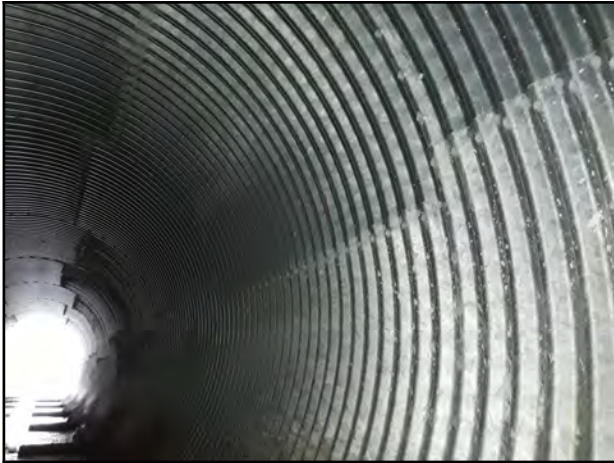
Photo 25 - Pipe wall from 7:00 o'clock to 5:00 o'clock in overall in excellent condition.
