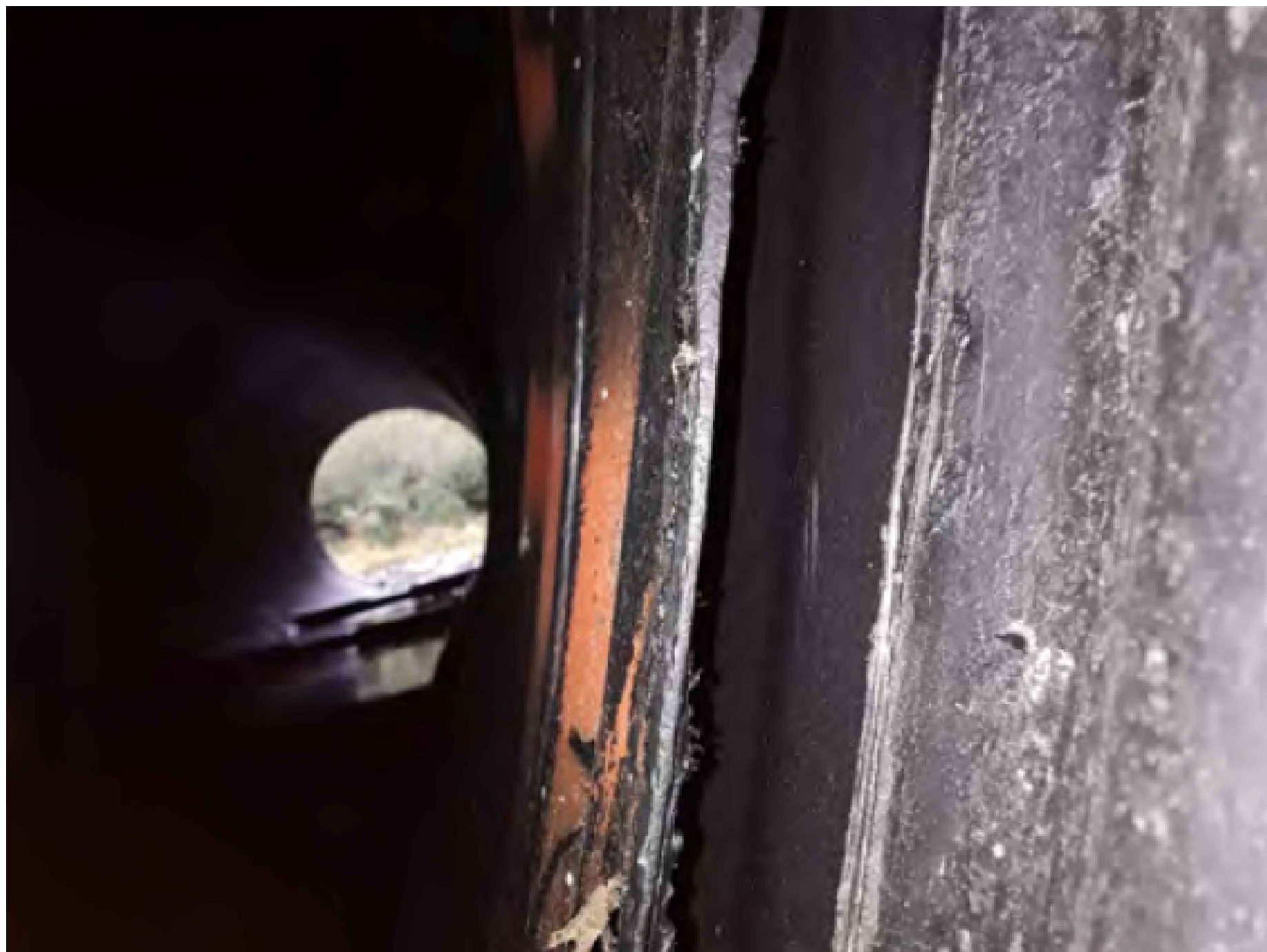
EXAMPLE PHOTO: V-3 OFFSET JOINT BY APPROXIMATELY 30mm WITH A VISIBLE COUPLER AND LEVEL 3 WATER INFILTRATION EVIDENT.
