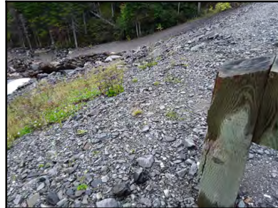
Photo 4 - Minor damage on post along outlet guardrail.
