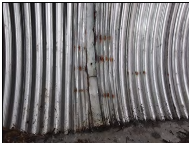
Photo 18 - V-1: Separated and offset joint by approximately 120 mm with visible backfill material, as well as surface corrosion at joint connection.
