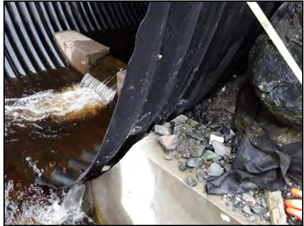
Photo 14 - Active water flowing between pipe wall and outlet headwall, with a separation of approximately 40 mm.
