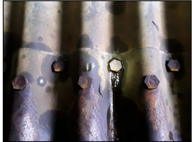
Photo 32 - V-2: Level 3 water infiltration at bolt.
