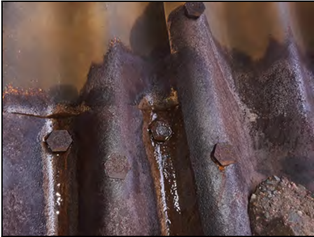
Photo 31 - V-1: Level 3 water infiltration at seam.
