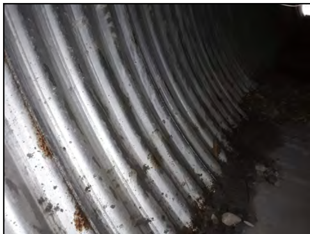
Photo 14 - Typical surface corrosion present throughout the pipe.
