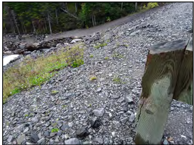
Photo 4 - Minor damage on post along outlet guardrail.
