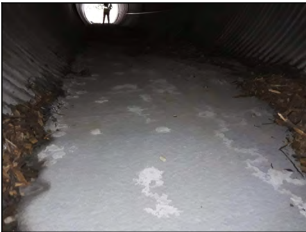
Photo 27 - Pipe was previously lined with a concrete paved invert.
