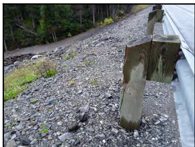
Photo 7 - Minor damage to post along the outlet guardrail.
