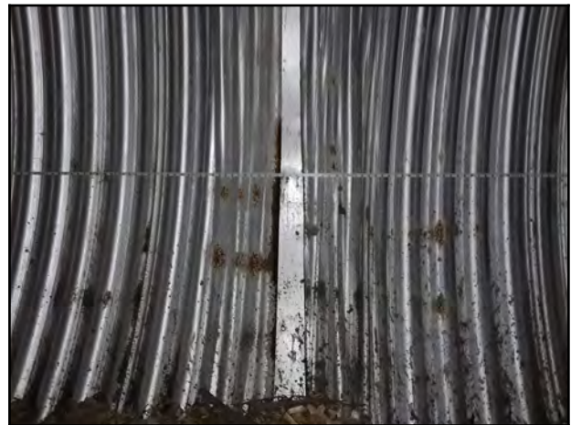
Photo 22 - V-2: Separated and offset joint by approximately 110 mm with visible filter fabric, and backfill material present.
