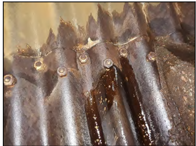
Photo 40 - V-10: Level 3 water infiltration at bolt.
