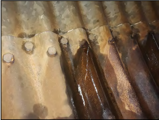
Photo 37 - V-7: Level 3 water infiltration at bolt.
