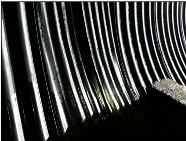
Photo 33 - V-5: Offset joint by approximately 50 mm with a visible coupler.
