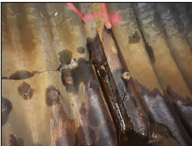
Photo 35 - V-5: Level 3 water infiltration at seam.
