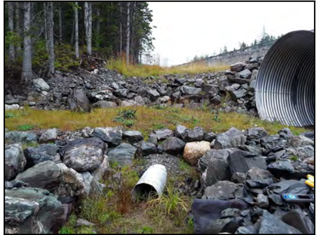
Photo 26 - Ditch drainage CMP pipe located upstream of the asset.
