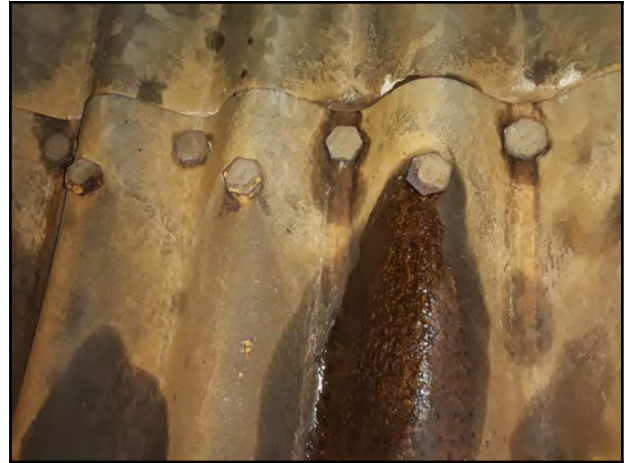
Photo 38 - V-8: Level 2 water infiltration at bolt.
