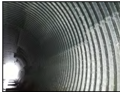
Photo 25 - Pipe wall from 7:00 o'clock to 5:00 o'clock in overall in excellent condition.
