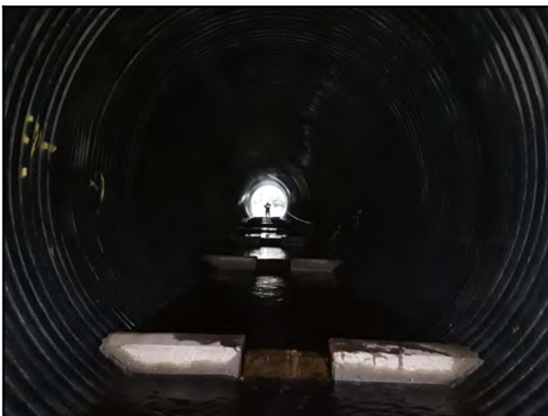
Photo 23 - Upstream pipe alignment and shape.
