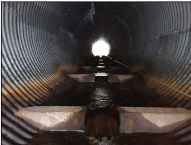
Photo 27 - Pipe has a total of 15 fish weirs installed.
