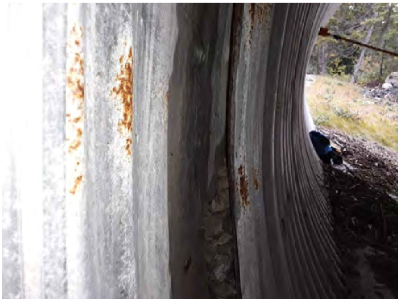
EXAMPLE PHOTO: V-J SEPARATED AND OFFSET JOINT BY APPROX. 120mm WITH VISIBLE BACKFILL MATERIAL AS WELL AS SURFACE CORROSION AT JOINT CONNECTION
