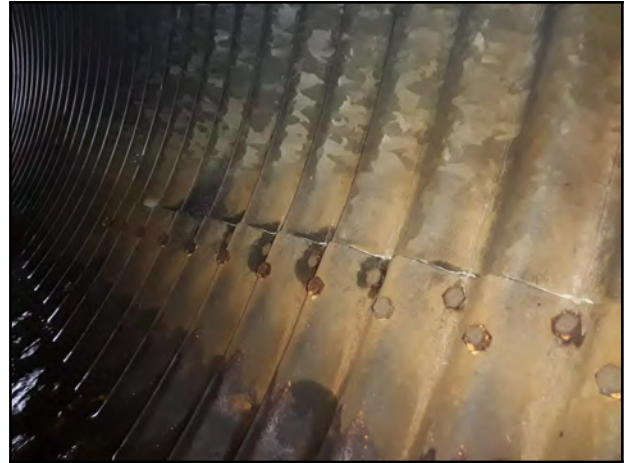
Photo 26 - Typical level 1 water infiltration at bolts along the seams at the 5:00 o'clock position.
