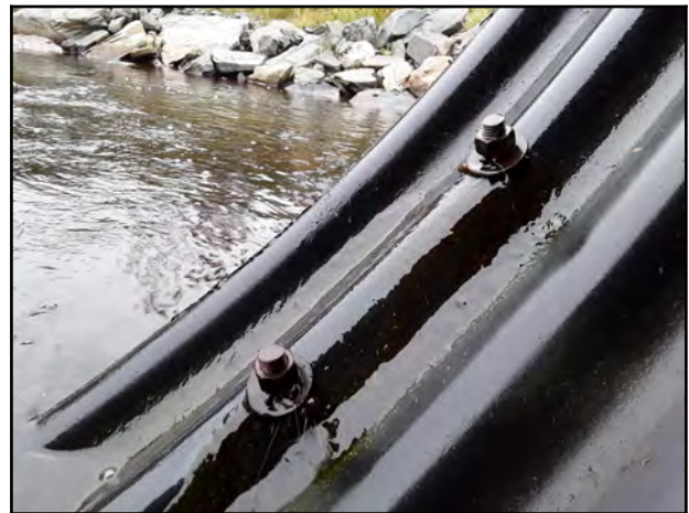
Photo 34 - V-6: Level 3 water infiltration at bolts.
