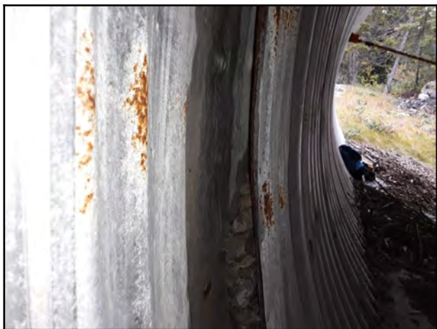
Photo 17 - V-1: Separated and offset joint by approximately 120 mm with visible backfill material, as well as surface corrosion at joint connection.
