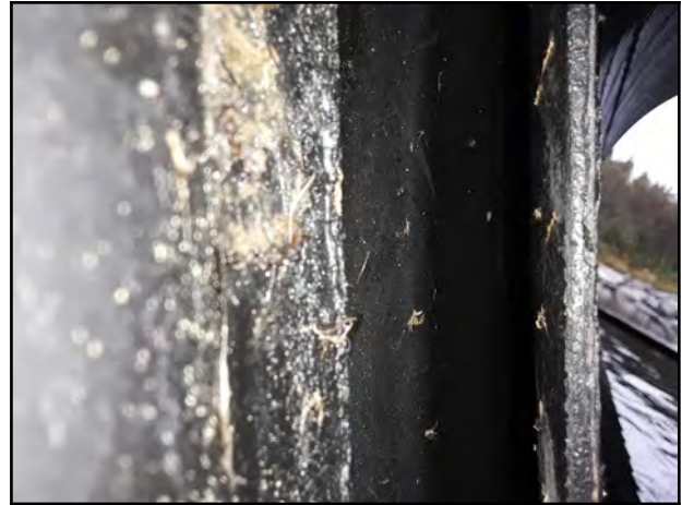
Photo 32 - V-5: Offset joint by approximately 50 mm with a visible coupler.
