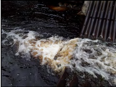
Photo 20 - Pipe outlet is perched by approximately 700 mm in height.
