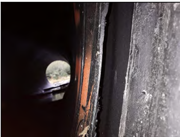
Photo 29 - V-3: Offset joint by approximately 30 mm with a visible coupler and level 3 water infiltration evident.
