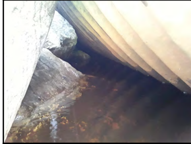
Photo 22 - Water pooling along the north side of the inlet pipe wall.
