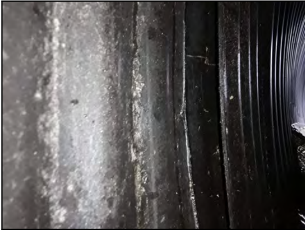
Photo 25 - V-1: Offset joint by approximately 40 mm with a visible coupler.
