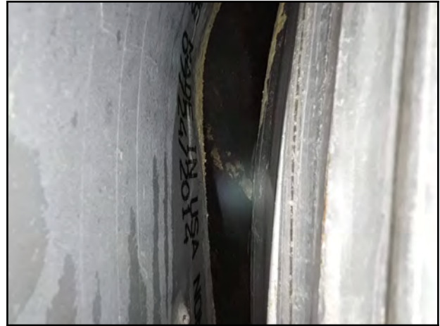
Photo 20 - V-2: Separated and offset joint by approximately 110 mm with visible filter fabric, and backfill material present.
