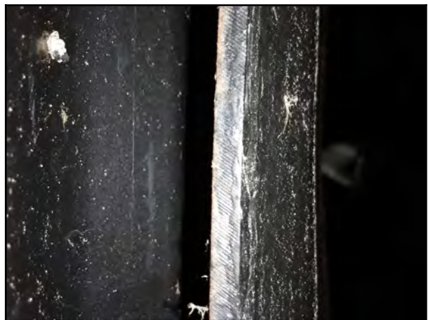
Photo 30 - V-4: Separated and offset joint by approximately 60 mm with a visible coupler.
