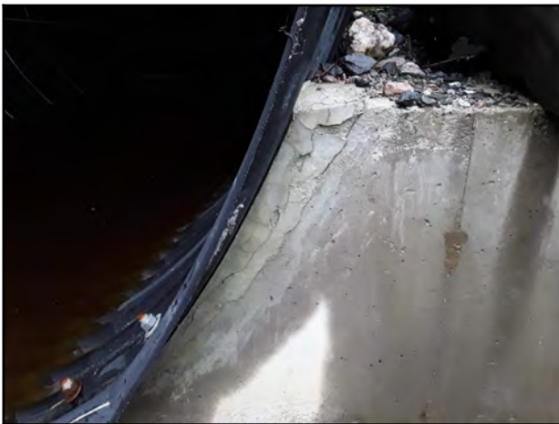
Photo 15 - Minor spalling along the inlet headwall.
