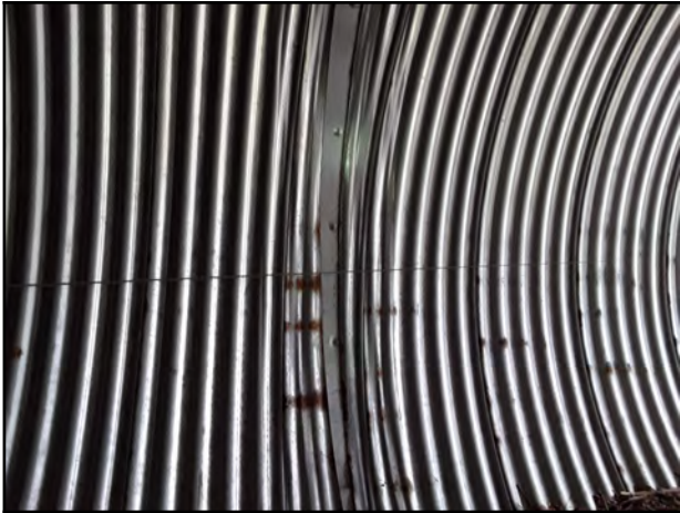
Photo 25 - V-3: Separated joint by approximately 120 mm with a visible coupler.
