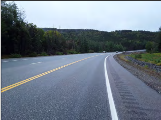
Photo 1 - West approach has a moderate downhill vertical grade with a long right-hand horizontal curve.
