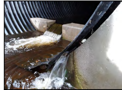
Photo 13 - Active water flowing between pipe wall and outlet headwall, with a separation of approximately 40 mm.
