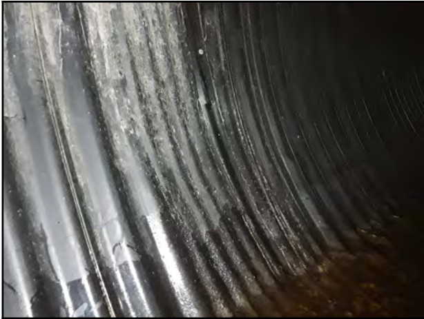
Photo 31 - V-4: Separated and offset joint by approximately 60 mm with a visible coupler.
