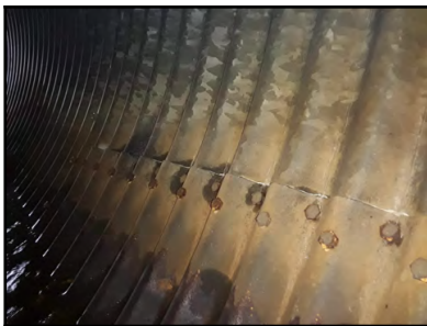
Photo 26 - Typical level 1 water infiltration at bolts along the seams at the 5:00 o'clock position.
