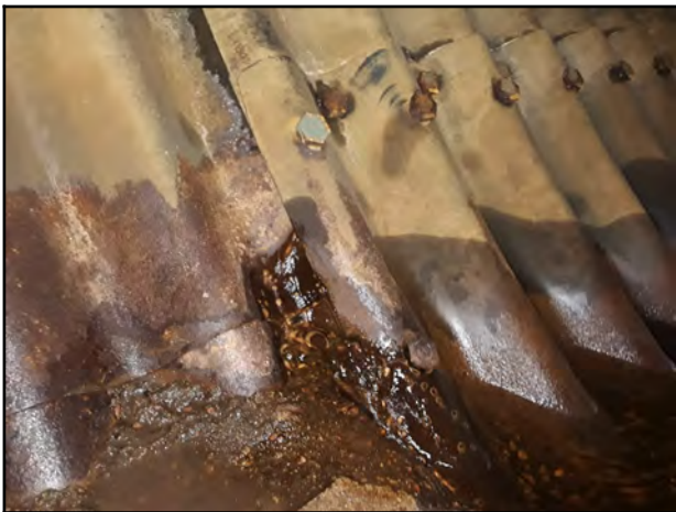
Photo 39 - V-9: Level 3 water infiltration at bolt and seam.
