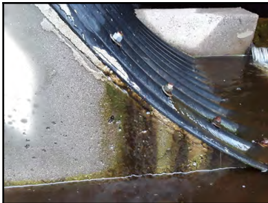
Photo 12 - Active water flowing between headwall and pipe wall at the outlet.
