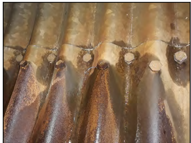
Photo 36 - V-6: Level 3 water infiltration at bolt.
