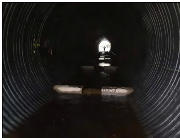
Photo 40 - Pipe had a total of 9 fish weirs placed approximately 5.00 m apart.
