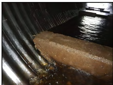
Photo 18 - Typical water flow between fish weirs and pipe wall.
