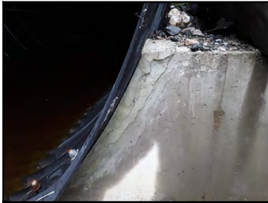
Photo 15 - Minor spalling along the inlet headwall.
