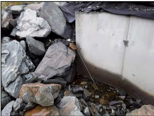
Photo 21 - Water pooling along the outlet concrete headwall.
