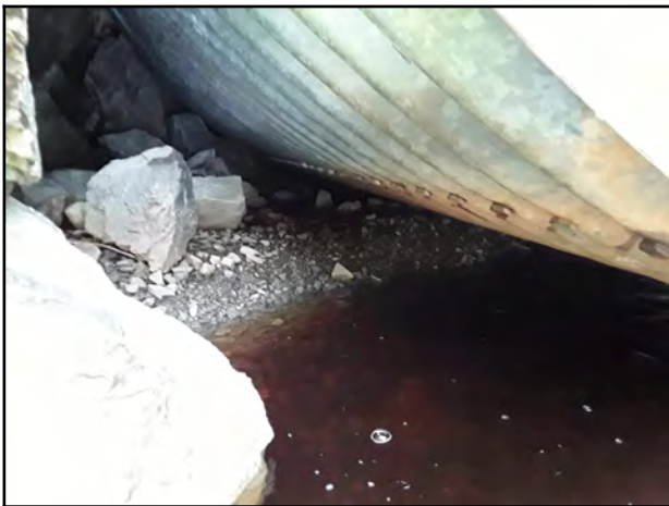
Photo 21 - Scouring measuring approximately 4100 mm in depth at the outlet.
