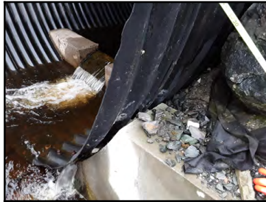
Photo 14 - Active water flowing between pipe wall and outlet headwall, with a separation of approximately 40 mm.
