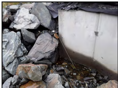
Photo 21 - Water pooling along the outlet concrete headwall.
