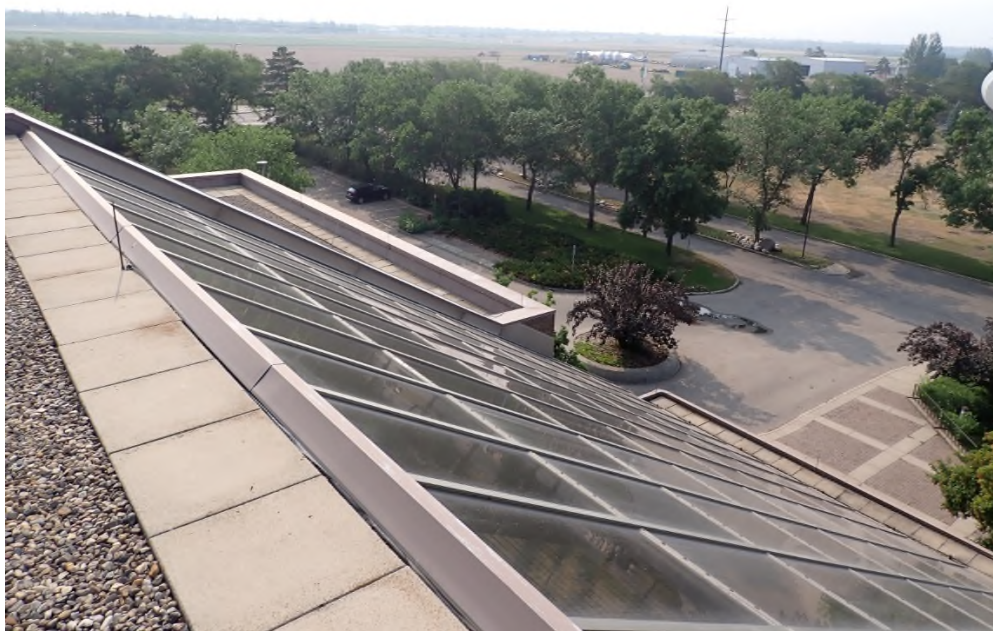
Photo 4 – Overview at the top transition of roof to the sloped glazing.
