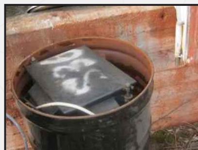
Sawmill Bay: Transformer containing PCBs
