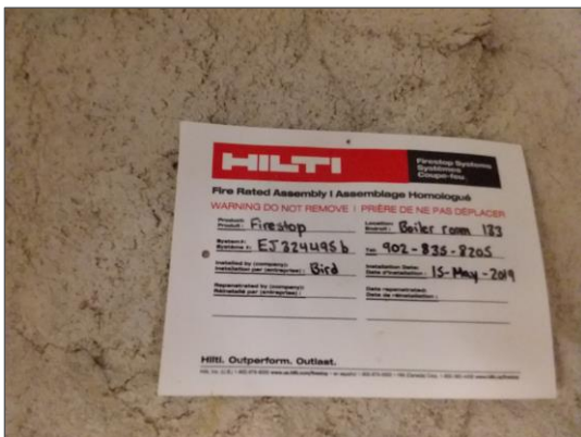
Spray fireproofing signage placed during firestop install
