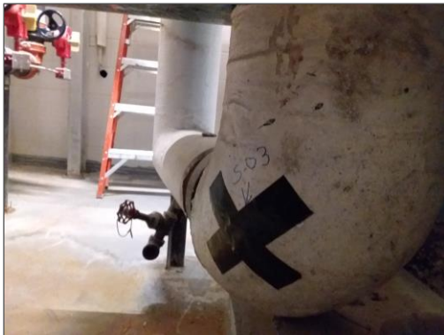
View of Boiler #2 pipe elbow sample location (S003)
