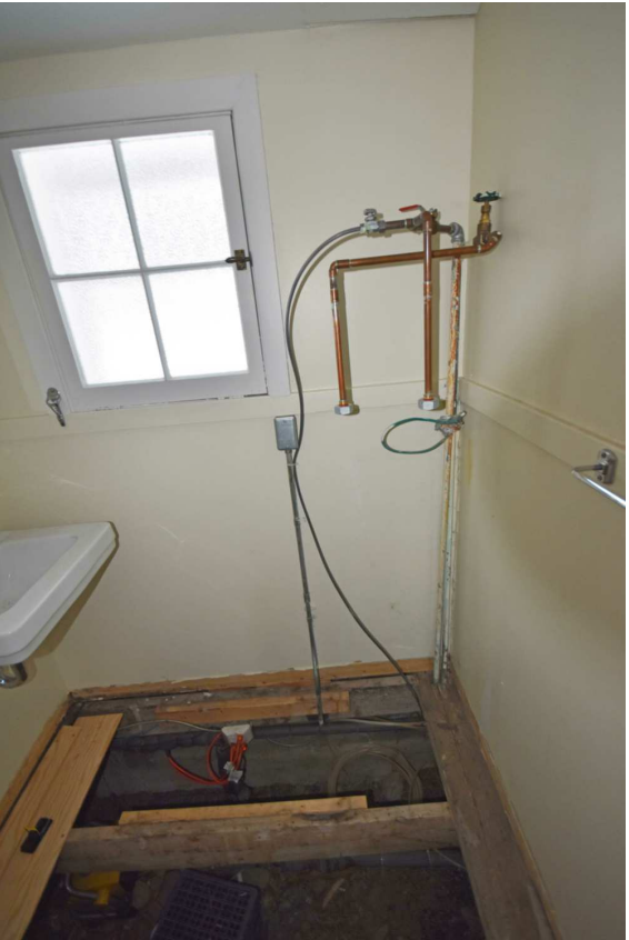
NORTH WASHROOM - REMOVE EXISTING HOT WATER HEATER PLUMBING
