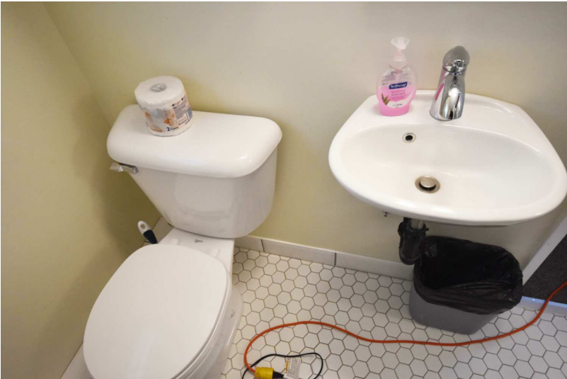
50mmx50mm HEXAGON MOSAIC FLOOR TILE 300mmx100mm BASE TILE REINSTALLED W/C AND LAVATORY
