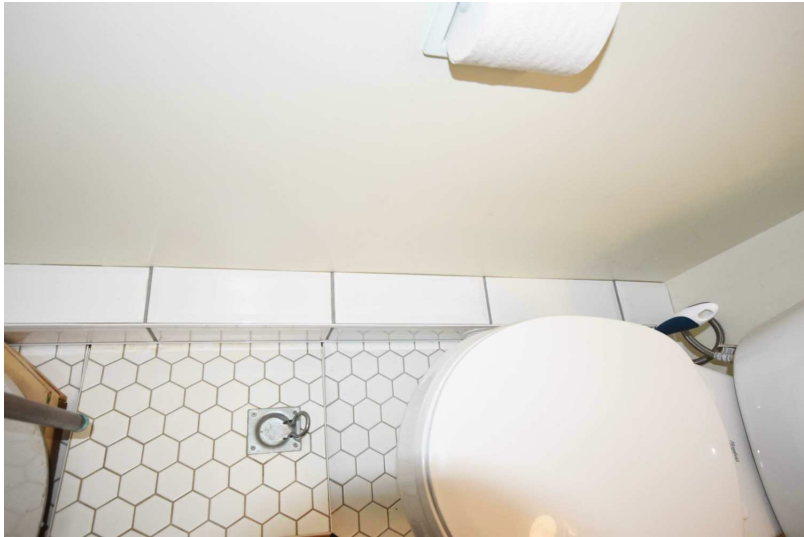
300mmx100mm BASE TILE 50mmx50mm HEXAGON MOSAIC FLOOR TILE FLOOR ACCESS HATCH AND 50mmx50mm FLOOR TILE ON TOP
