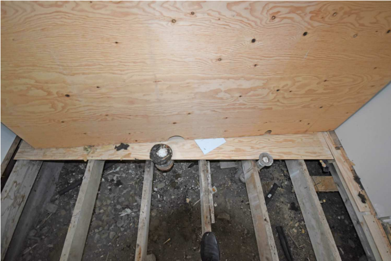
SOUTH WASHROOM - EXISTING WATER CLOSET AND SHOWER DRAINAGE
