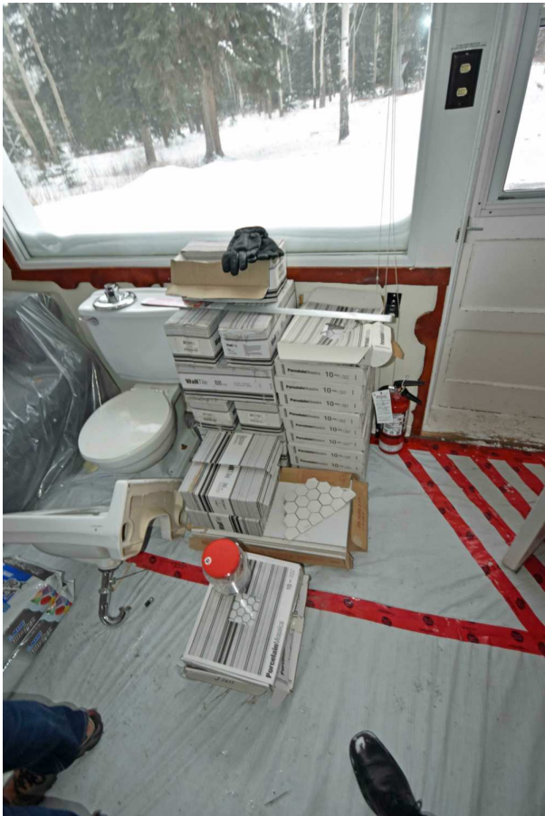
150mmx75mm SHOWER SURROUND TILE 10.5 BOXES WITH 88 TILES/BOX 300mmx100mm BASE TILE. 3 BOXES WITH 30 TILES/BOX 25mmx25mm HEXAGON MOSAIC SHOWER BASE TILE 50mmx50mm HEXAGON MOSAIC FLOOR TILE 10 BOXES WITH 88SQFT/BOX
