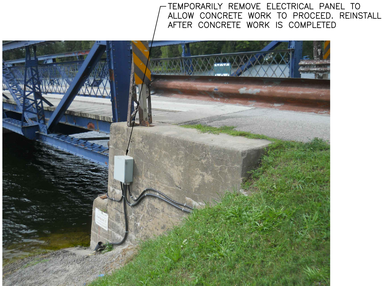
ELECTRICAL PANEL SOUTH ABUTMENT N.T.S.
