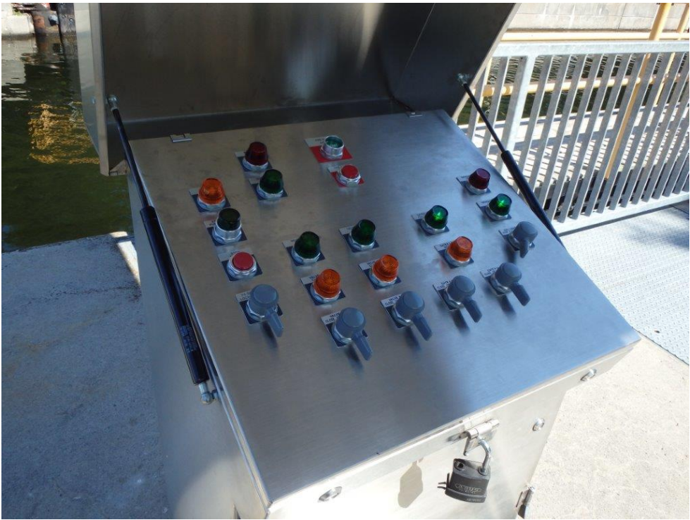
EXAMPLE OF CUSTOM COVER WITH GAS STRUTS
