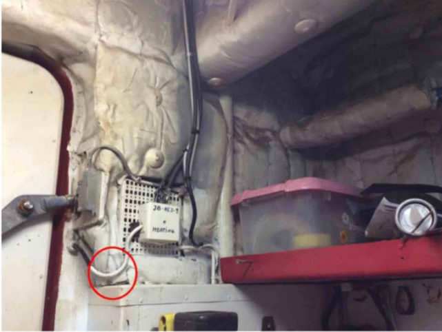
Material sample Welding Room — Wall — Canvas — Good — Asbestos-free material Chantal.Soulard - 2022-02-07 14:58
