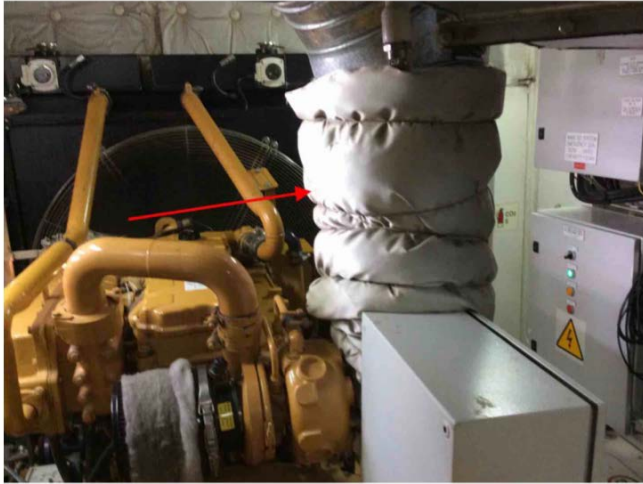
Material sample Generator Room — Pipe — Canvas — Good — Asbestos-free material Chantal.Soulard - 2022-02-07 15:06
