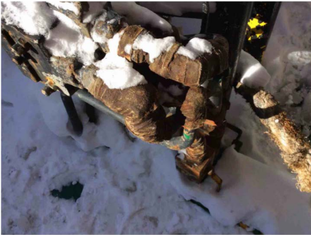
Material sample Outdoor — Equipment — Canvas — Good — Asbestos-free material Chantal.Soulard - 2022-02-07 16:36
