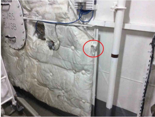
1 Material sample Bow Thruster Room — Wall — Canvas — Good — Asbestos-free material Chantal.Soulard - 2022-02-07 14:54
