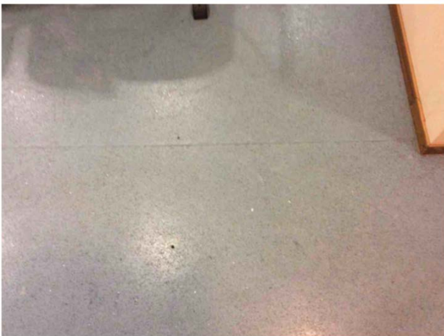
9 Material sample Main Room — Floor — Vinyl Tile — Good — Asbestos-free material Chantal.Soulard - 2022-02-07 15:11
