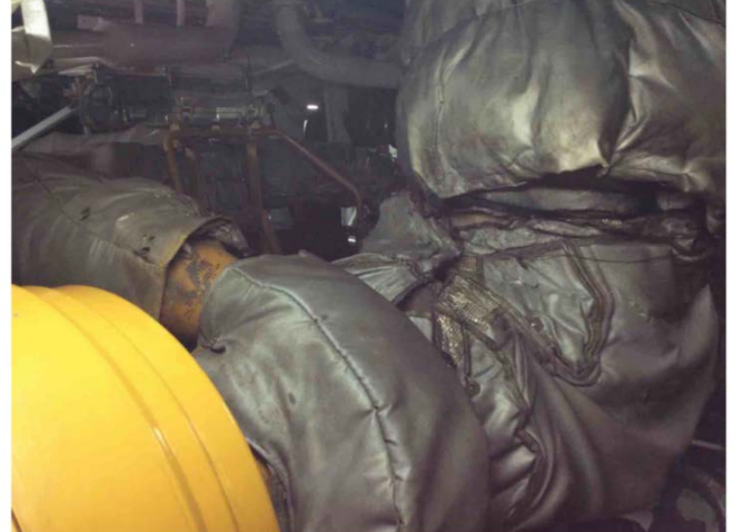
Material sample Engine Room — Pipe — Canvas — Fair — Asbestos-free material Chantal.Soulard - 2022-02-07 16:24
