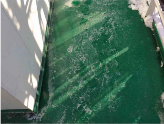
29 Paint sample Outdoor — Floor — Green — Good — Lead-free paint Chantal.Soulard - 2022-02-07 16:03
