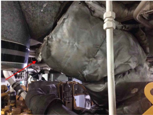
2 Material sample Engine Room — Pipe — Canvas — Fair — Asbestos-free material Chantal.Soulard - 2022-02-07 14:56
