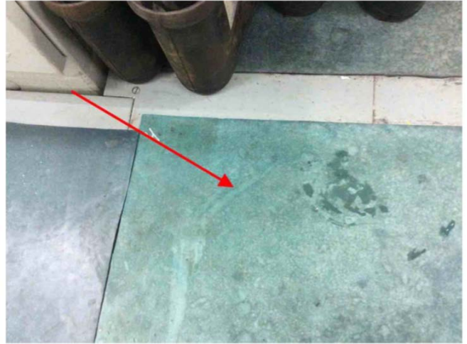
Material sample Switchboard Room — Floor — Rubber Mat — Good — Asbestos-free material Chantal.Soulard - 2022-02-07 16:49
