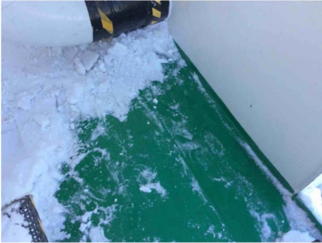
37 Paint sample Outdoor — Floor — Green — Good — Lead-free paint Chantal.Soulard - 2022-02-07 16:17
