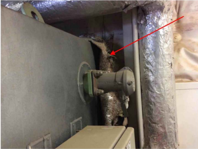
Material sample Incinerator Room — Pipe — Canvas — Fair — Asbestos-free material Chantal.Soulard - 2022-02-07 15:00
