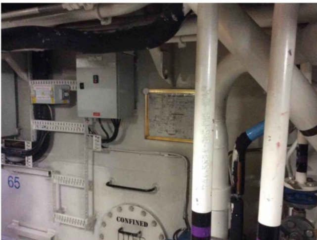
19 Paint sample Engine Room — Wall, ceiling and pipe — White — Good — Lead-free paint Chantal.Soulard - 2022-02-07 15:30
