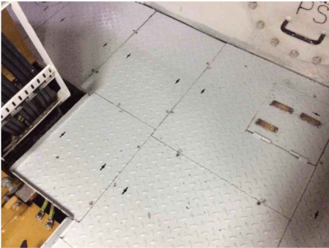
18 Paint sample Engine Room — Floor — Gray — Good — Lead-based paint Chantal.Soulard - 2022-02-07 15:28
