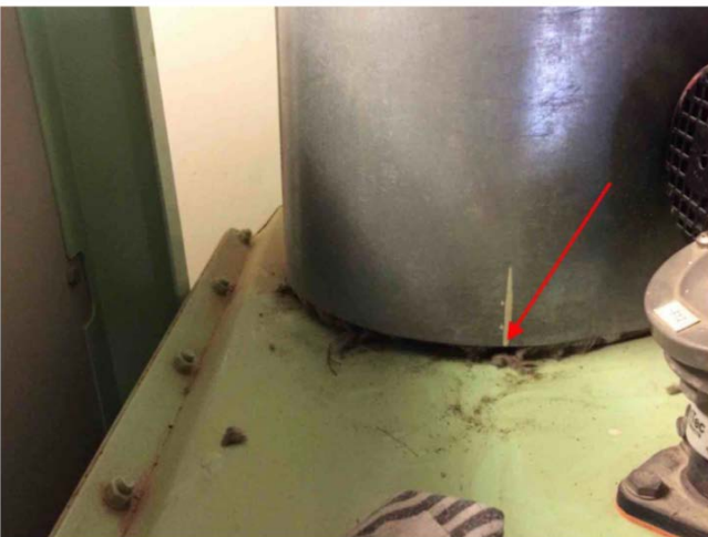
43 Material sample Incinerator Room — Pipe — Insulating Wool — Good — Asbestos-free material Chantal.Soulard - 2022-02-07 16:31
