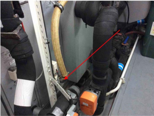
6 Material sample AC Room — Pipe — Canvas — Good — Asbestos-free material Chantal.Soulard - 2022-02-07 15:04
