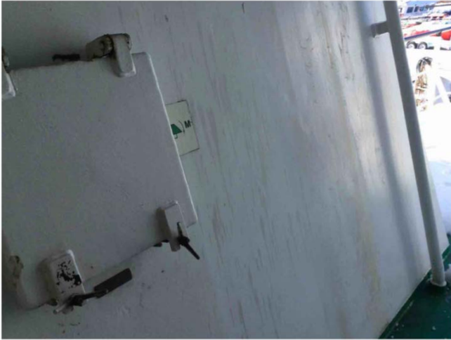
35 Paint sample Outdoor — Wall — White — Good — Lead-free paint Chantal.Soulard - 2022-02-07 16:13
