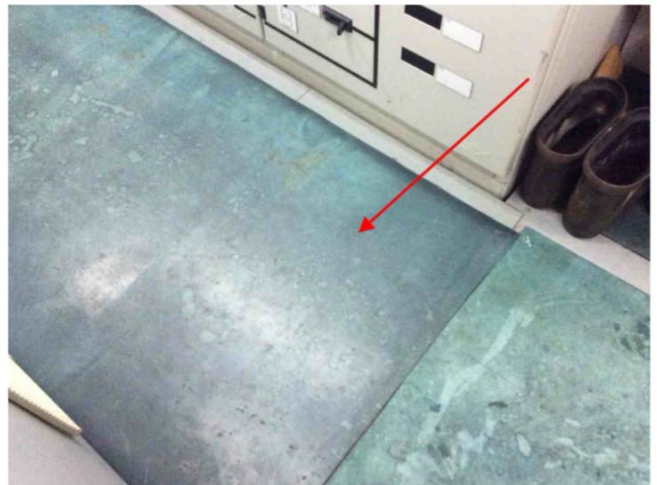
Material sample Switchboard Room — Floor — Rubber Mat — Good — Asbestos-free material Chantal.Soulard - 2022-02-07 16:50
