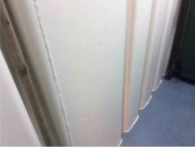
27 Paint sample Air Lock — Wall — White — Good — Lead-free paint Chantal.Soulard - 2022-02-07 15:59
