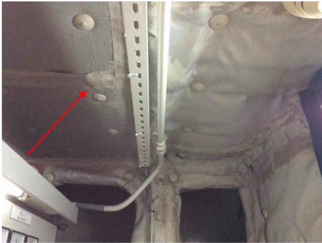
Material sample Generator Room — Ceiling — Canvas — Good — Asbestos-free material Chantal.Soulard - 2022-02-07 15:07
