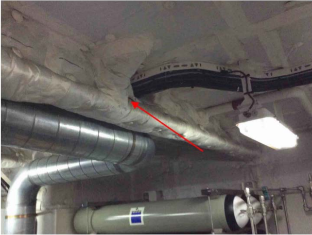
5 Material sample AC Room — Ceiling — Canvas — Good — Asbestos-free material Chantal.Soulard - 2022-02-07 15:02
