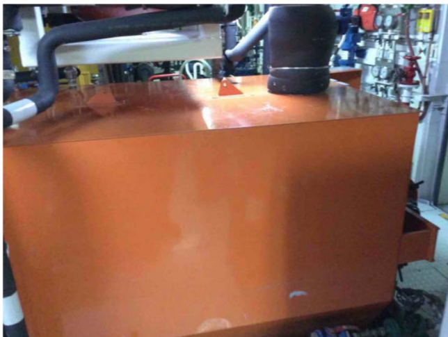
16 Paint sample Engine Room — Equipment — Orange — Good — Lead-based paint Chantal.Soulard - 2022-02-07 15:24
