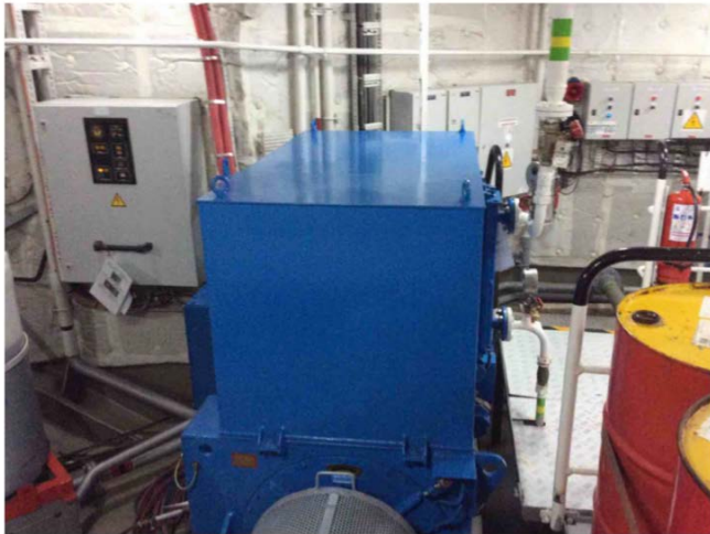
14 Paint sample Bow Thruster Room — Equipment — Blue — Good — Lead-based paint Chantal.Soulard - 2022-02-07 15:21
