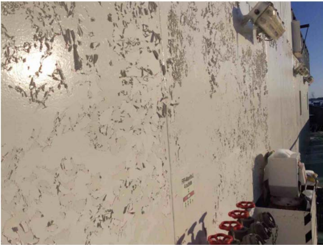
30 Paint sample Outdoor — Wall — White — Poor — Lead-free paint Chantal.Soulard - 2022-02-07 16:05
