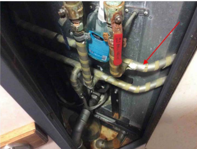
49 Material sample Tank — Pipe — Canvas — Good — Asbestos-free material Chantal.Soulard - 2022-02-07 16:52
