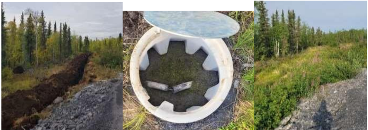
Figure 4: View of Typical Pull Box, Trenching and Naturalization
