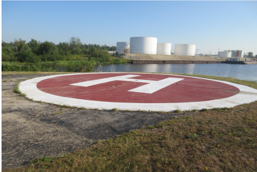
Signature - Exterior Helicopter Pad
