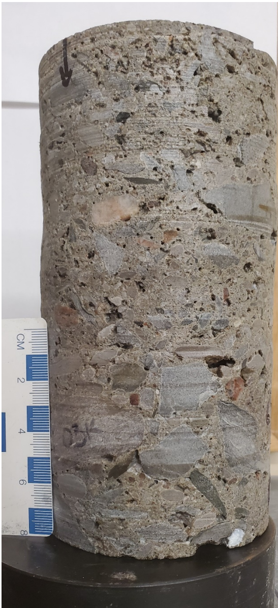
Photo 3A – Core No. 3 Pre-Compression
