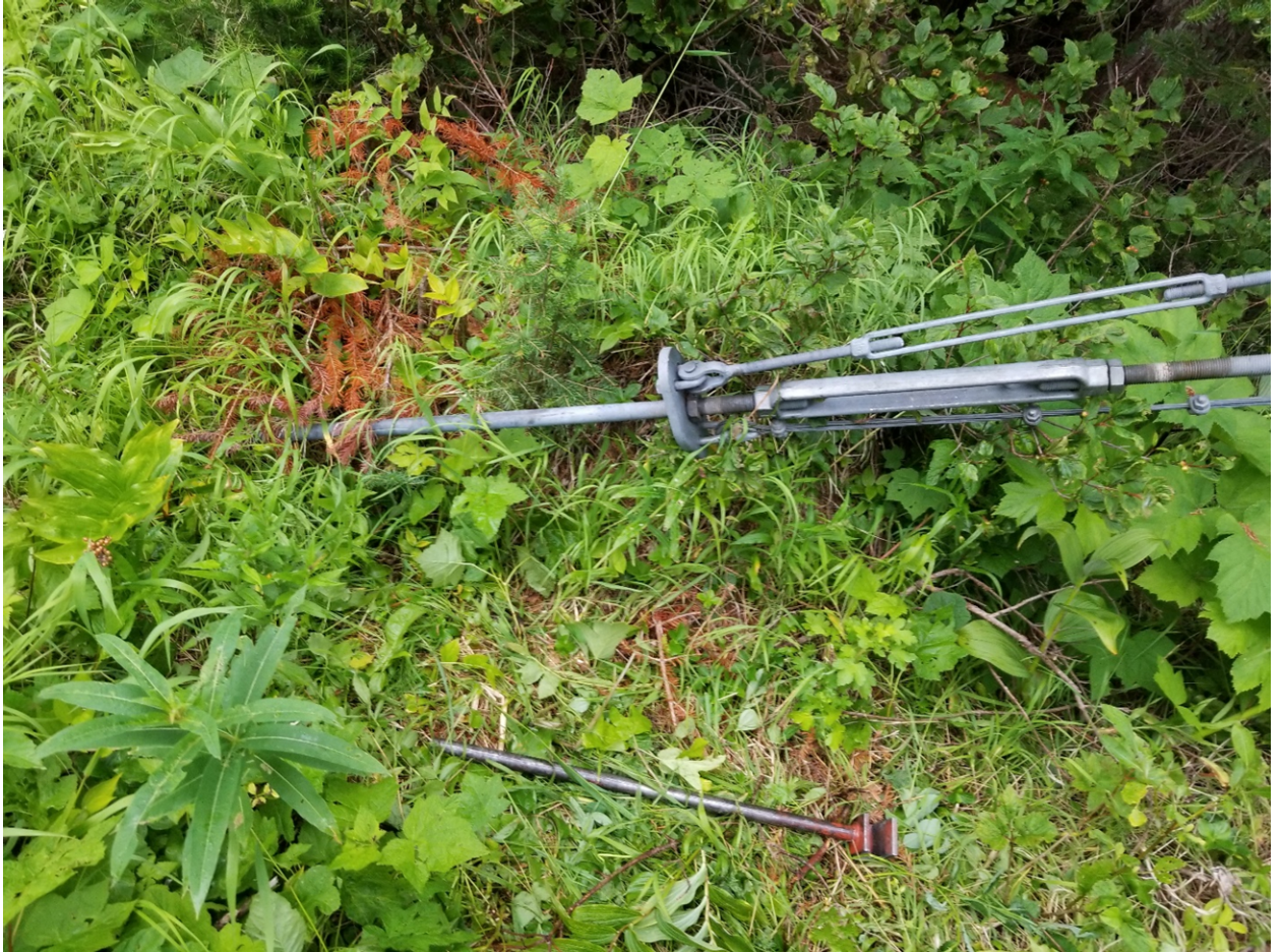
Photo 7: Left Bank Home-Side Anchor Connection
