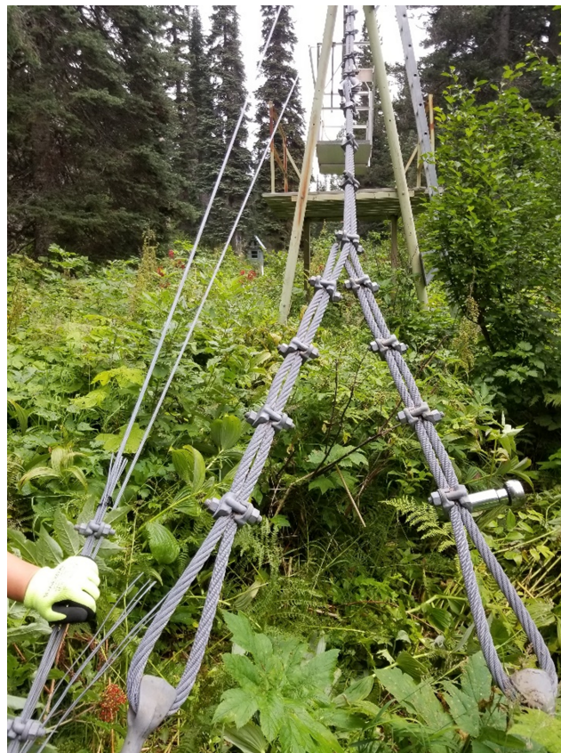
Photo 2: Right Bank Far-Side Bridle Cable
