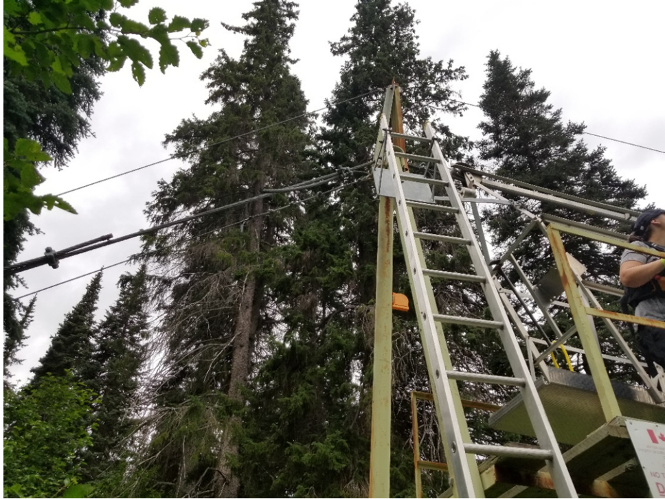
Photo 3: Right Bank Far-Side Top of A-Frame
