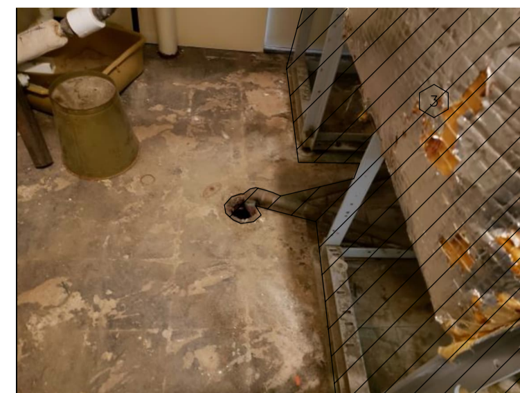
PHOTO NO.3 – EXISTING AUTOCLAVES AND PIPING REMOVAL (3)
