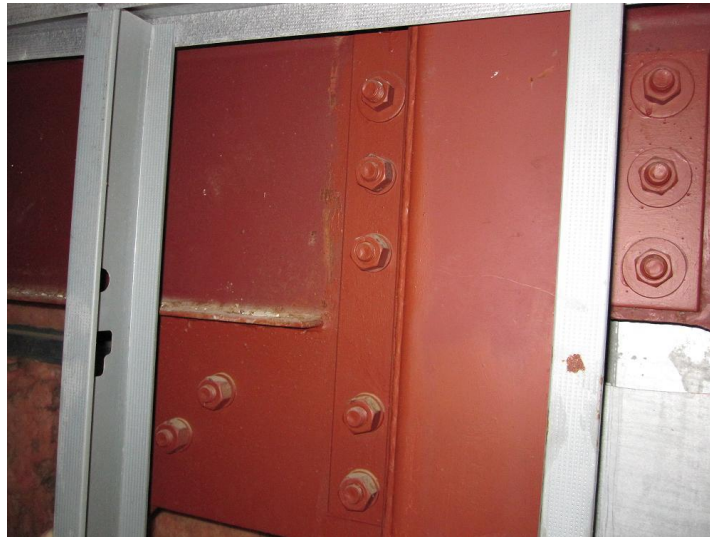
Photograph 5 - : Structural Steel Column and Connection
