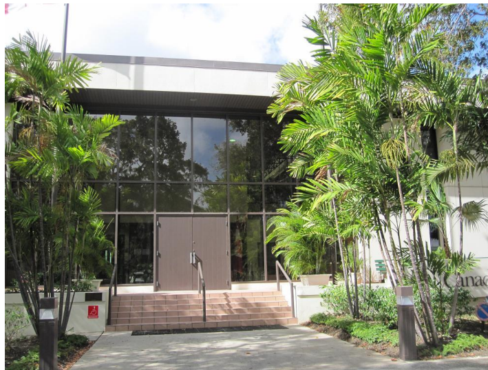
Photograph No. 8 - Exterior Façade
