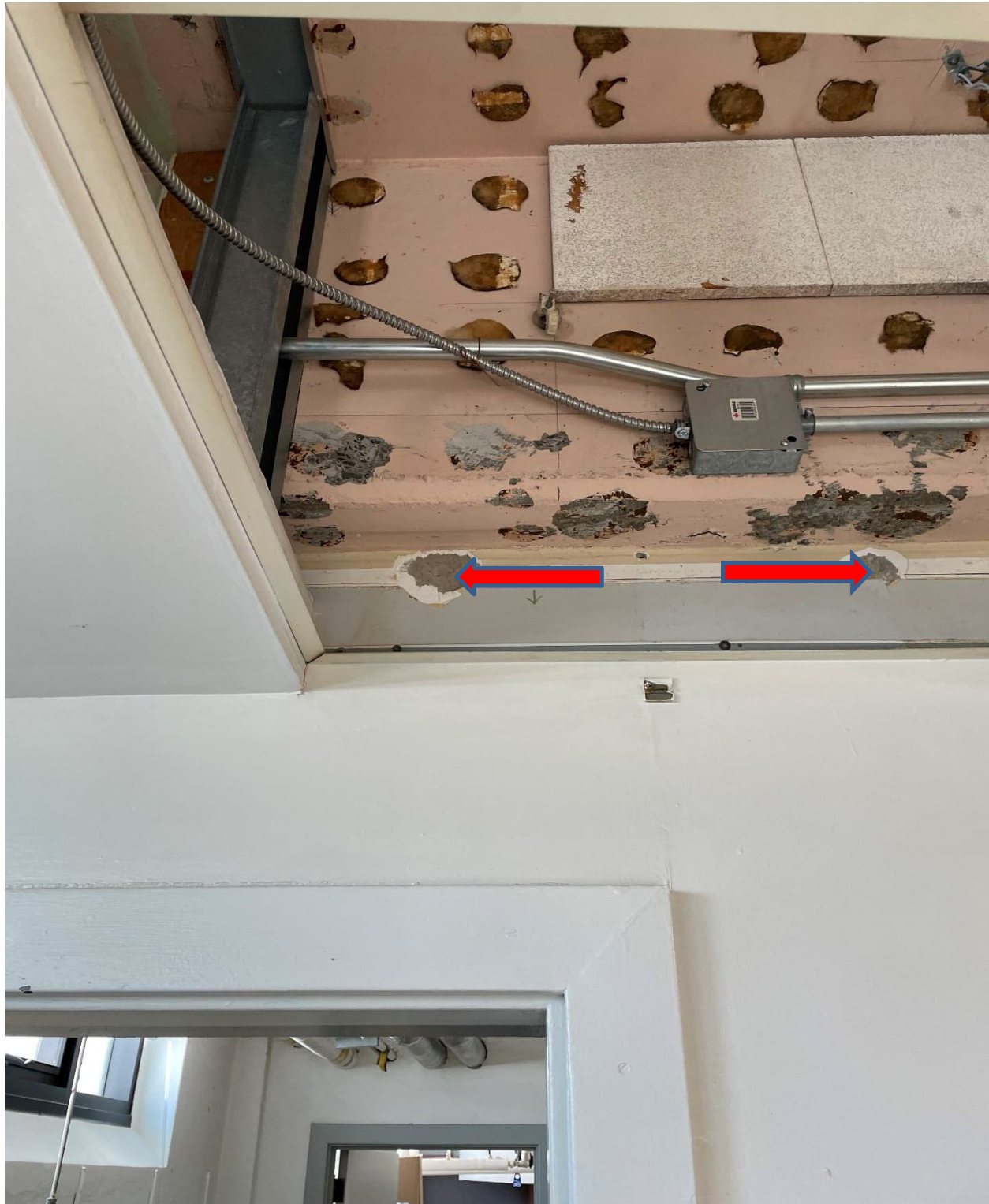
Photo 2: Asbestos-containing plaster dividing wall in Room 066 contains 1% Chrysotile asbestos (Sample 08-A (Grey layer)). 30 cm x 30 cm Stick-on Ceiling Tile and Mastic were confirmed to be non-asbestos.
