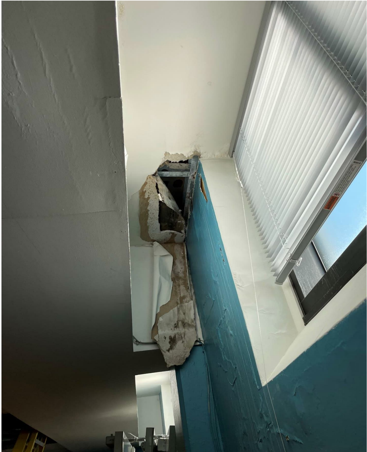
Photo 1: Asbestos-containing Skim Coat on Concrete perimeter Wall (wall with windows) contains 1% Chrysotile asbestos (Sample ID 02C). This material is water damaged here. Mould (Sample M-01) was also confirmed on the drywall bulkhead here.
