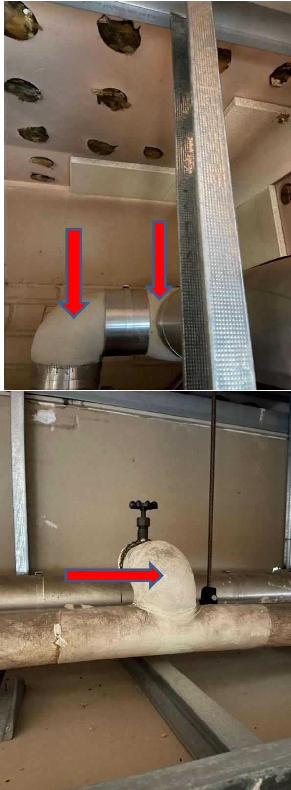
Photos 3&4: Asbestos-containing pipe fitting insulation on pipes contains 40% Chrysotile asbestos (Sample 06)
