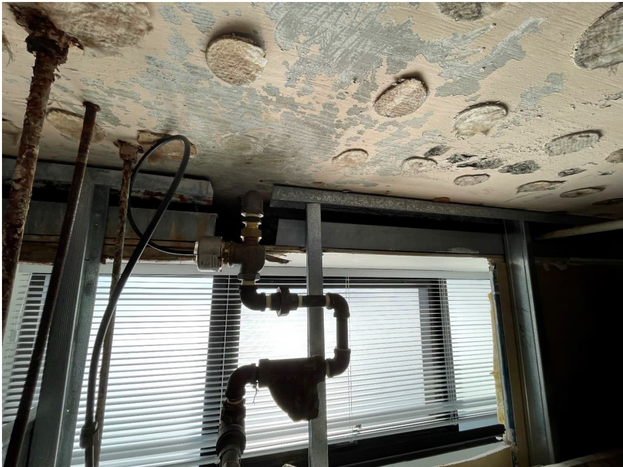
Photo 7: Pink paint on the concrete deck was confirmed to contain 491 ppm lead (LP01). Plaster walls and ceilings were confirmed to be non-asbestos. Vinyl baseboard mastic and the 12" x 12" vinyl floor tiles and associated mastic were all confirmed to be non-asbestos as well.
