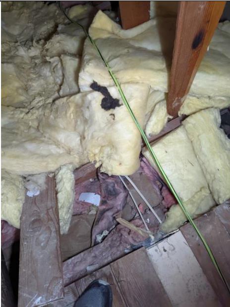
Sample: 38686 - 11 Location: Building 12 - Attic Description: Insulation Asbestos: None Detected
