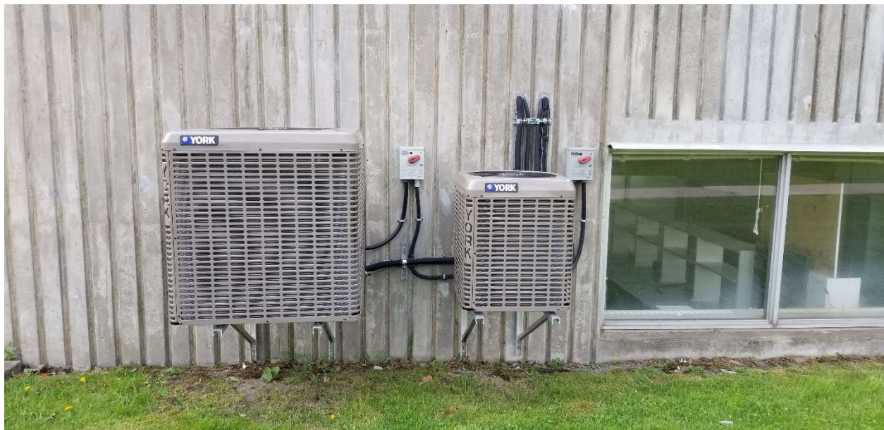
Photograph 9: External air handling units, confirmed to contain 10 lbs of R410A halocarbons.
