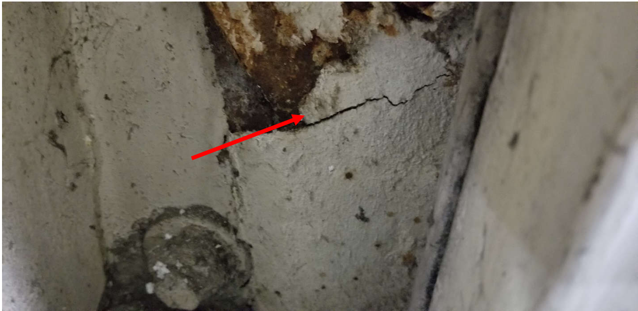
Photograph 3: Parging cement on the Penthouse perimeter wall was confirmed to contain 65% Chrysotile asbestos (Sample ID 41133-14A).
