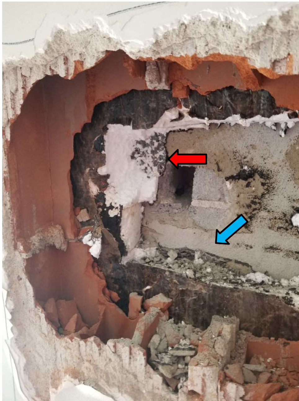
Photograph 5: Styrofoam, within the perimeter wall, contains tar layers on both sides. The tar on the exterior side (red arrow) contains 1% Chrysotile asbestos (Sample 41133-26A). Grey paring cement, within the perimeter wall (blue arrow), contains 1% Chrysotile asbestos (Sample 41133-21A[2]). To access the tar, demolition into the perimeter wall from the interior or exterior of the structure will be required. Materials are well adhered, whereby grinding, or mechanical means would be required for removal.
