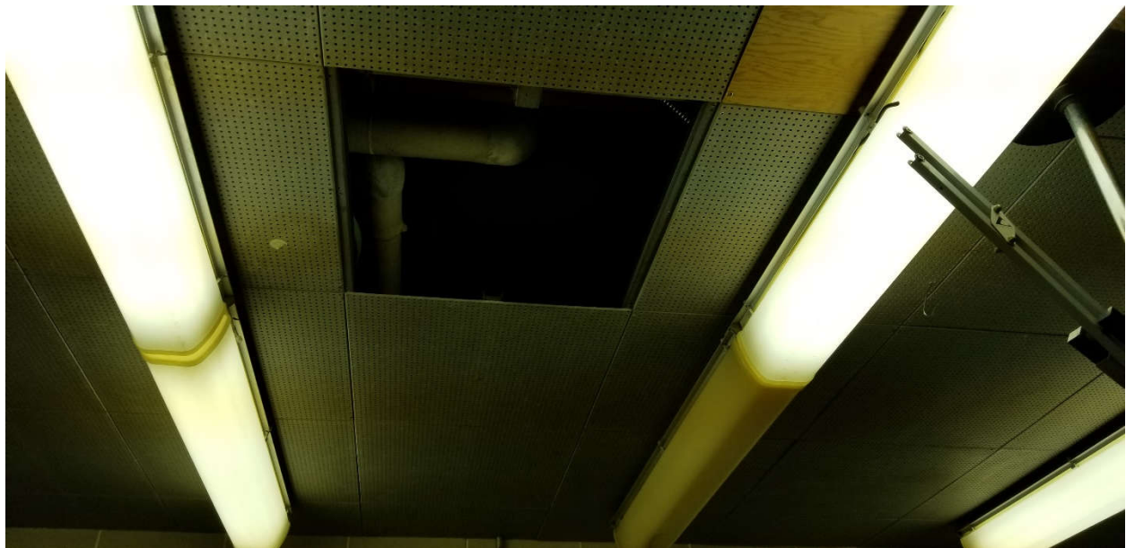
Photograph 2: Transite ceiling panels, observed in Room B88, were confirmed to contain 15% Chrysotile asbestos (Sample ID 41133-05A)
