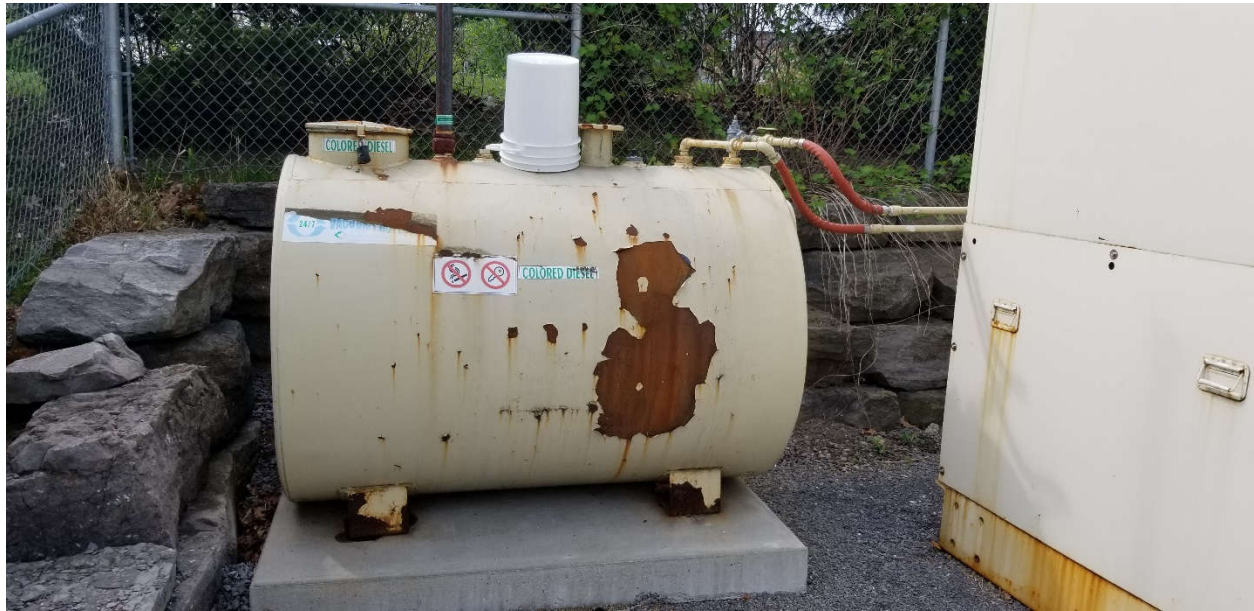
Photograph 8: A diesel storage tank, with an estimated capacity of 7,500L, was observed on the exterior, eastern side of the building.
