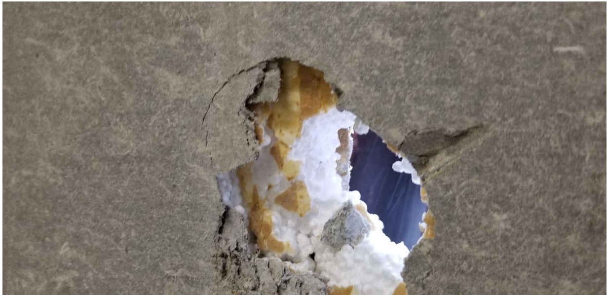
Photograph 1: Transite panels, observed in the penthouse, were confirmed to contain 15% Chrysotile asbestos (Sample ID 41133-06A)
