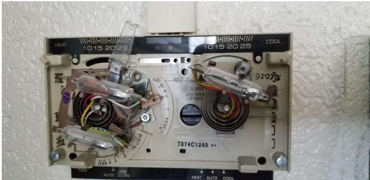
Photograph 6: Thermostats, containing glass ampules of mercury, were observed throughout the building.
