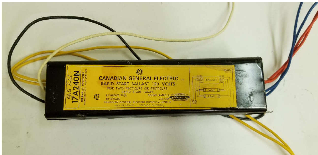
Photograph 7: PCB ballasts were observed within the building.
