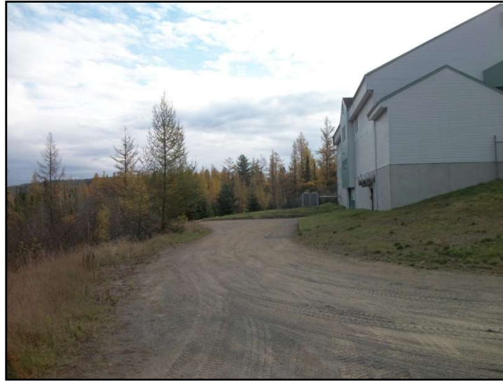
Access to Door No. 10
