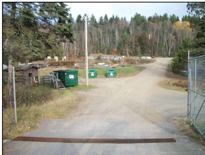
Access to containers
