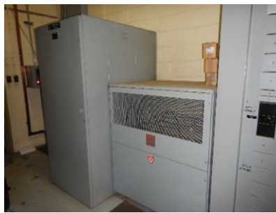
CSB Emergency Distribution (across from normal CSB, transformers on either side of distribution panel)
