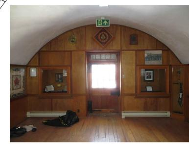
ARTIFACTS TO BE REMOVED AND STORED BY CLIENT. THE PANELING AND FRAMING OBTAINING WINDOWS RW2-26 & 27 IS TO BE CAREFULLY REMOVED TO ALLOW FOR THE RESTORATION OF THE WINDOWS AND DOOR AND RECONSTRUCTED AT JOB END.
