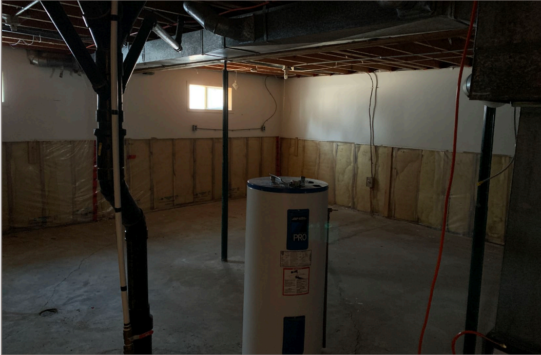
Photo 5: View of the common area of the basement, facing northwest. Note lower portions of drywall on the interior walls of the basement have been abated. There were no obvious signs of mould at the time of the HBMA.
