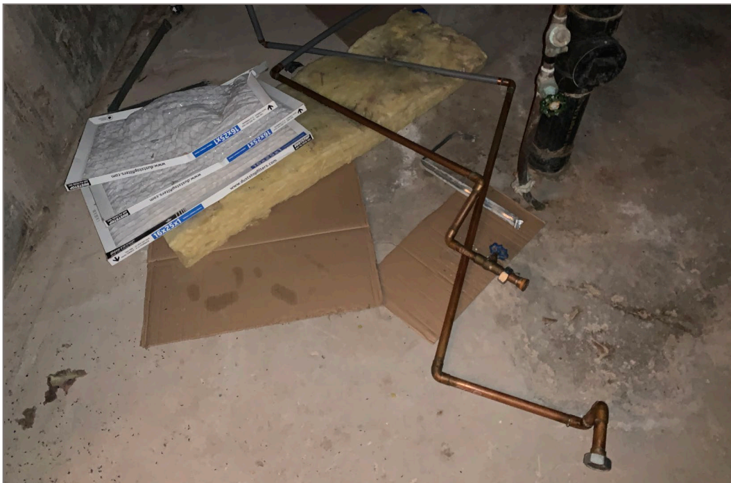
Photo 6: Copper piping observed in the basement at the time of the HBMA which may contain lead solder.
