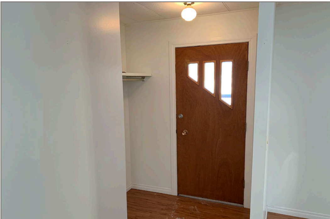
Photo 2: Interior of the front entrance of the subject building, facing north. Note white interior walls (P001) not found to be lead-based paint. Also note the drywall joint compound (DWJC) throughout the subject building, confirmed to contain asbestos.
