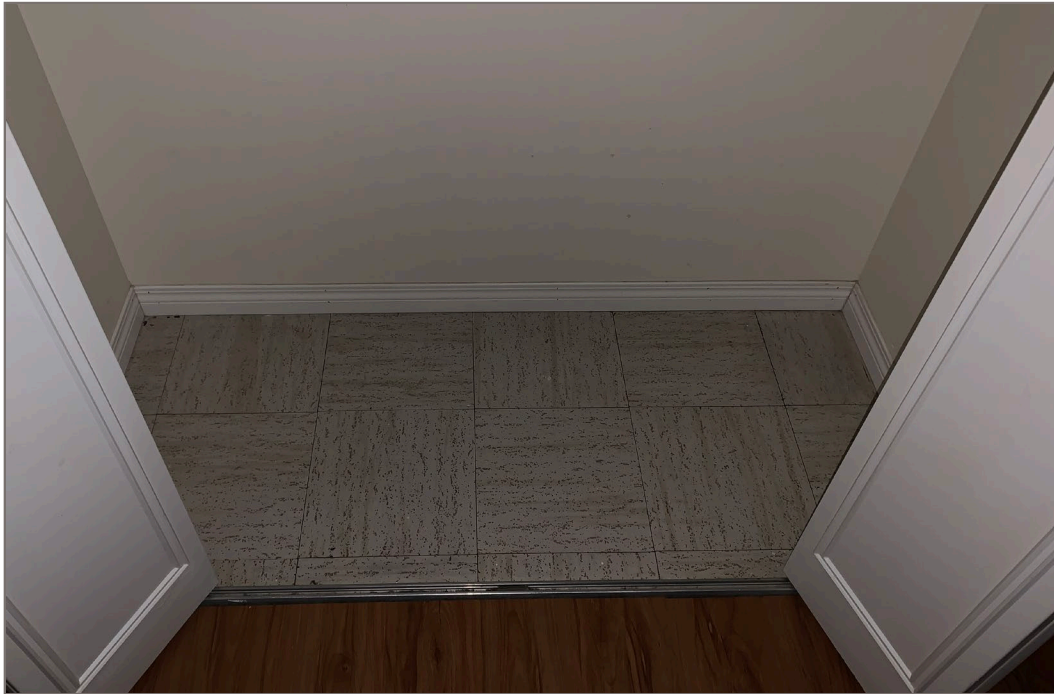
Photo 3: View of the grey vinyl floor tile (VFT01) observed in all closets throughout the main floor, as well as hidden below the engineered wood floor (FLOORING01) in bedroom 2. The vinyl floor tile was confirmed to contain asbestos.
