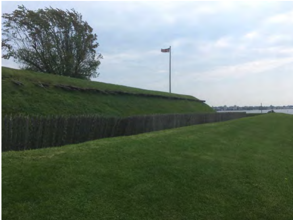
Figure 1 – West Palisade and Fraising, looking South (Sept-2017)
