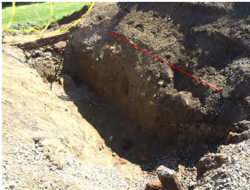
Figure 2 - Test pit on interior berm, excavated by others
