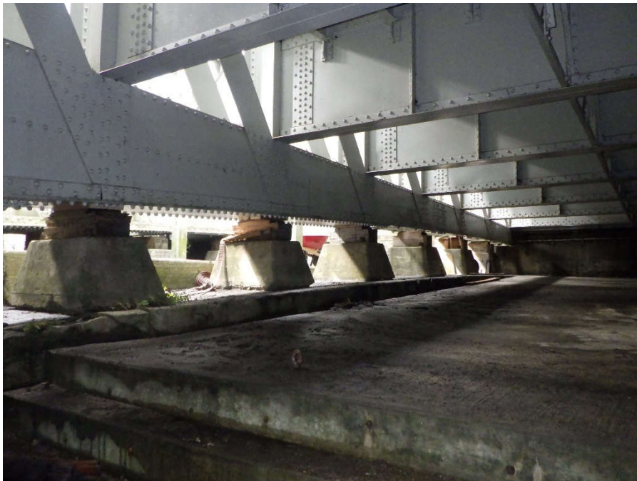
Photo 6. North Chamber Sitting on Rest Blocks.
