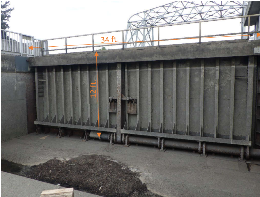
Photo 5. South Upper Reach Gate.
