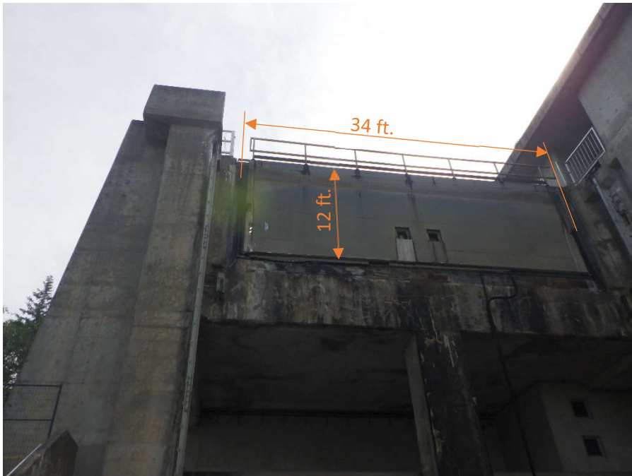
Photo 4. North Chamber Upper Reach Gate. Scale View of Gate.
