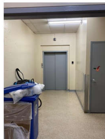
Picture 4: Picture from inside loading dock area Looking towards Freight elevator door
