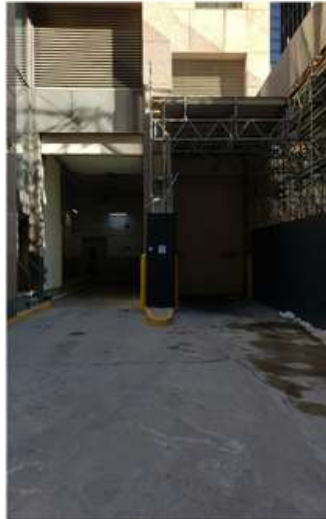
Picture 2: Loading dock 121 with door open
