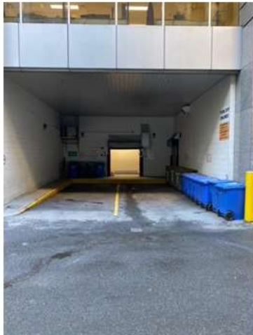
Picture 2: Loading dock 255 with door open
