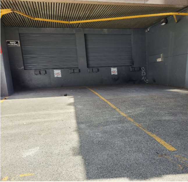
Picture of loading area
