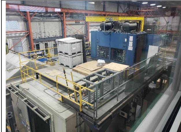
Photograph 5 - Top of Existing LEC (Compressor Package) 1
