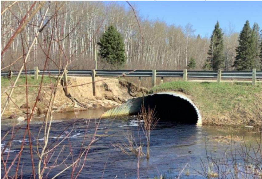
Km 26 carried two lanes of traffic over Jackfish Creek. Constructed in 1970, an elliptical multiplate corrugate steel pipe arch 5.550 m wide X 2.440 m high. X 11 m long was used with a CIP concrete headwall. Existing Condition Photo:
