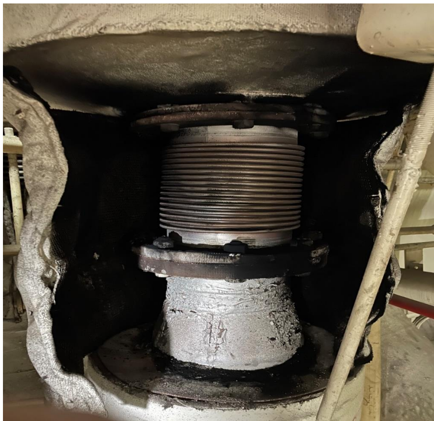
Figure 13.2.1 Existing Bellows
