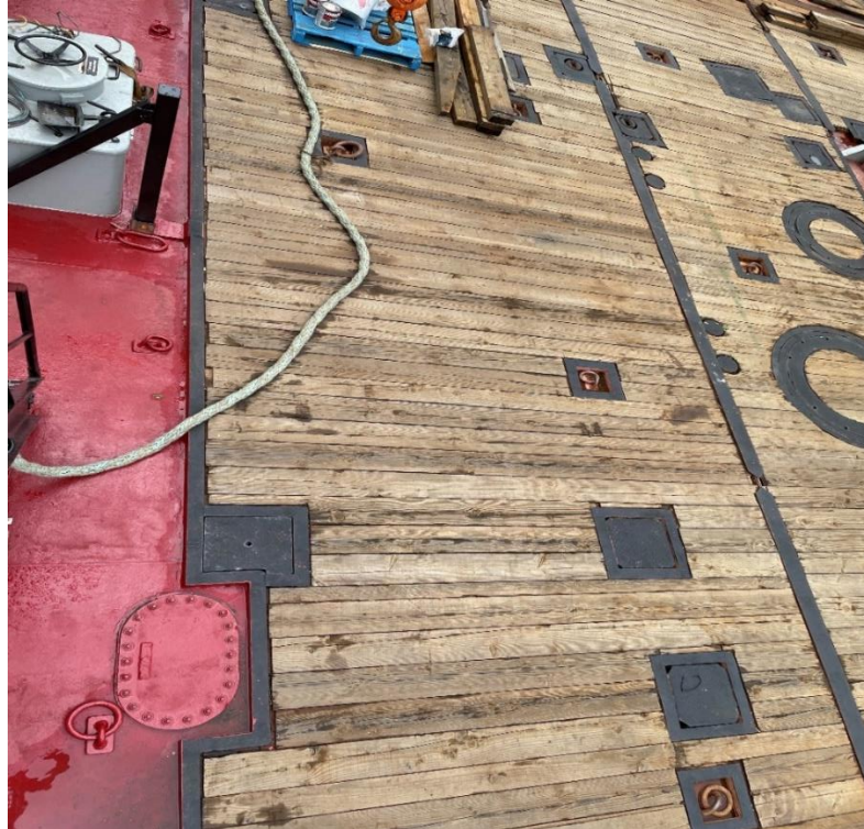
Figure 11.8-1 Wooden deck on the Main deck
