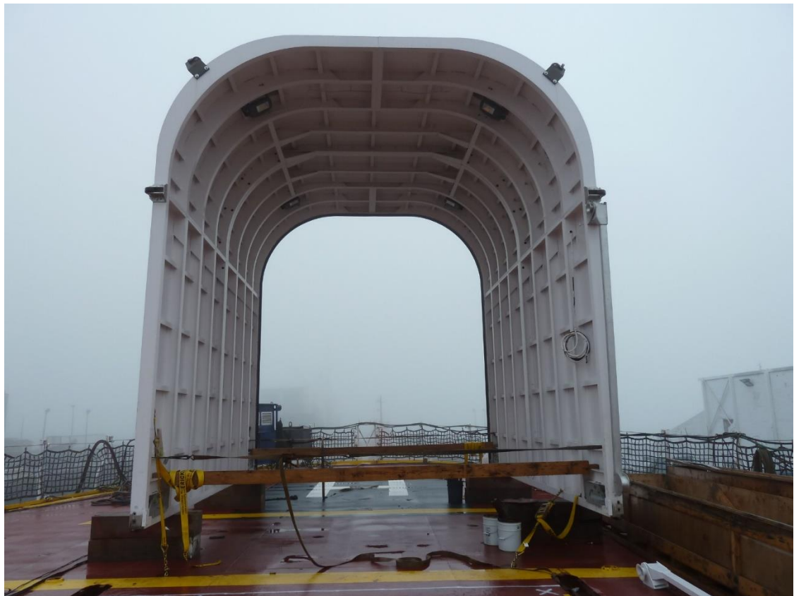
Figure 16.6.1-Photo of a section of the hanger ready for lifting
