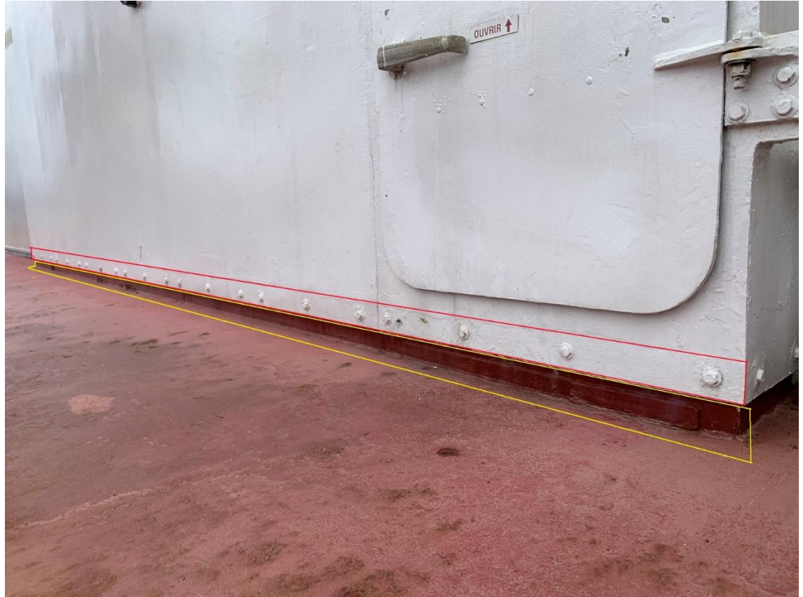
Figure 16.6.2- Steel and aluminum section to be replaced
