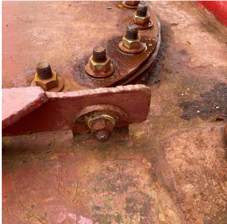
Figure 111.8-2 Anchorage of a retaining bar
