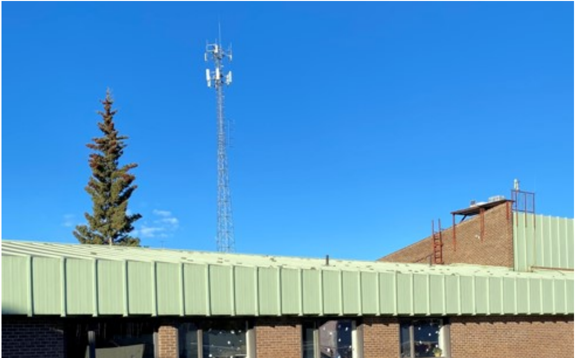
5.3 Rear of building Image 1
