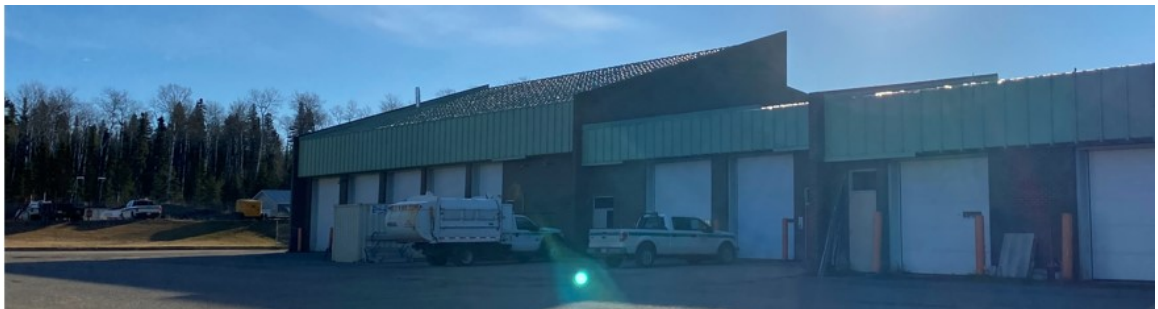
5.4 Rear of building Image 2
